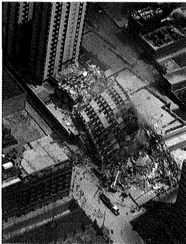
**Fig. 15-17** In 1985, buildings of intermediate height collapsed in Mexico City as a result of an earthquake far from the city. Taller and shorter buildings remained standing. (John T. Barr/Getty Images News and Sport Services)
