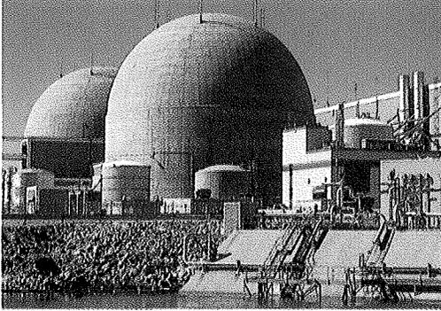
**Fig. 20-12** The North Anna nuclear power plant near Charlottesville, Virginia, which generates electric energy at the rate of 900 MW. At the same time, by design, it discards energy into the nearby river at the rate of 2100 MW. This plant and all others like it throw away more energy than they deliver in useful form. They are real counterparts of the ideal engine of Fig. 20-8. (© Robert Ustinich)
