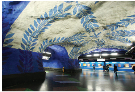
The bedrock through which the system in Stockholm is built has been made an architectural feature, and there are murals and quantities of art located everywhere throughout the system.
