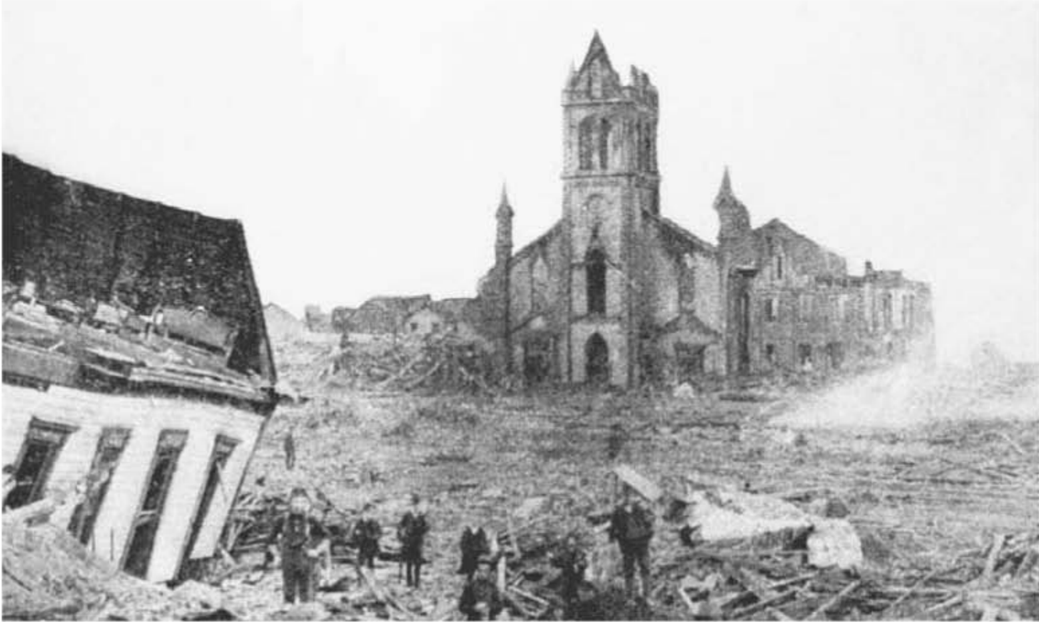
The aftermath of the Galveston hurricane of September 1900, which devastated coastal Texas. The tropical storm claimed more than 6,000 lives, making it the deadliest hurricane to ever hit the United States. NOAA
