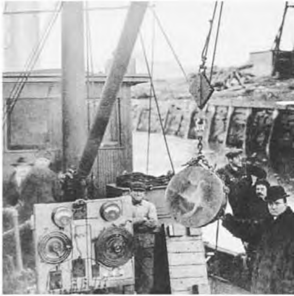
The Fessenden oscillator, shown in 1914 aboard the tugboat Susie D , was the first test of the sonic radar technology. The crew, headed by Robert Williams, was looking for icebergs, but they also found the ocean bottom. NOAA Central Library
