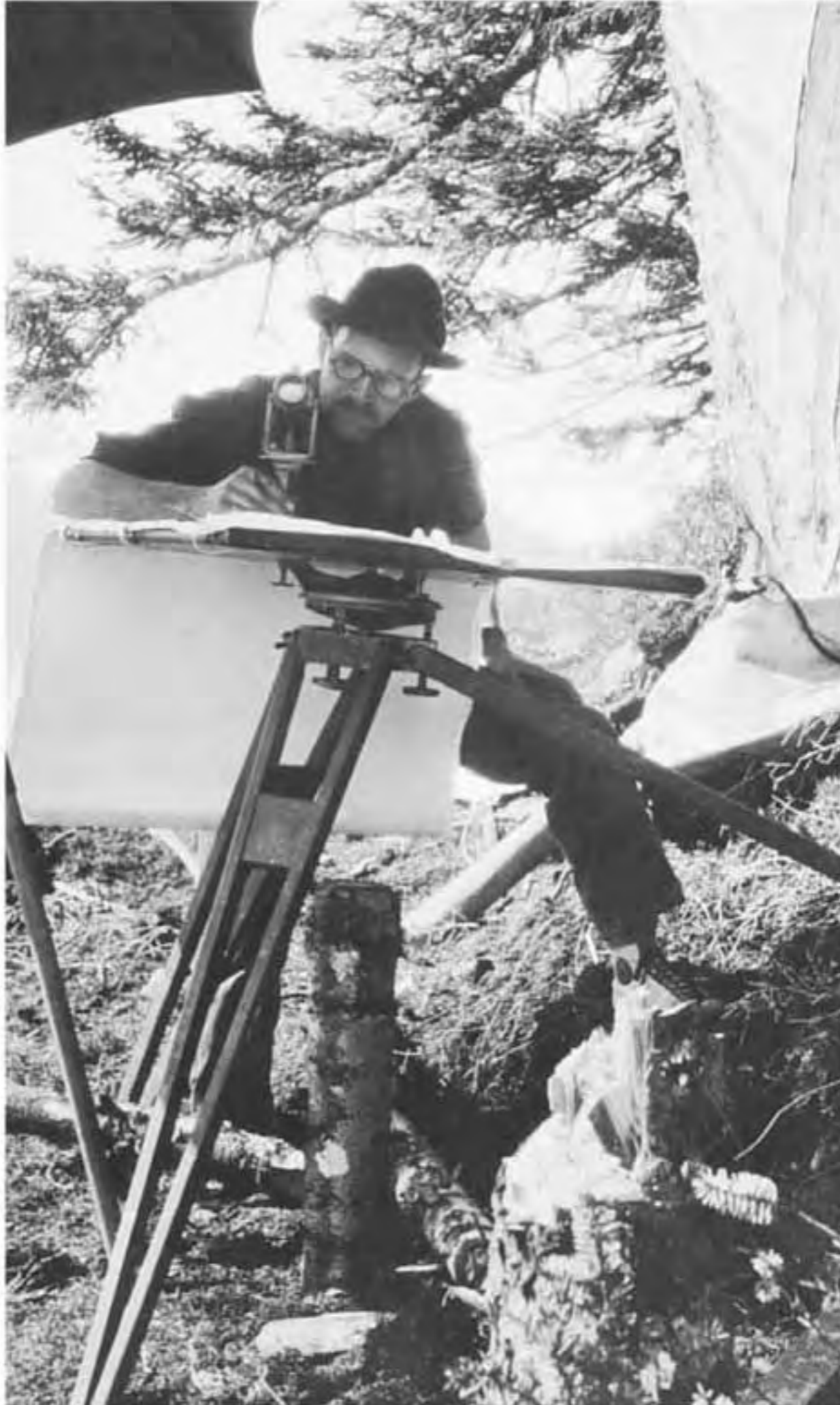
Oceanographic work can be varied: This plane table crew, at work on a 1928 survey on Alaska's Kenai Peninsula, was headed by NOAA Rear Admiral Paul Smith of the Coast & Geodesic Survey. NOAA/Family of Rear Admiral Paul A. Smith, C&GS
