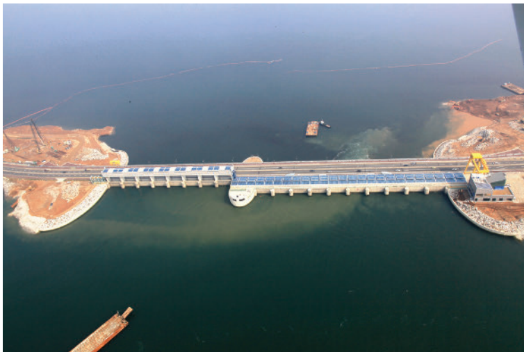
Figure 12.11 The Sihwa tidal power station in South Korea has a production capacity of 254 MW (see Table 12.3). Photograph provided by Dr Sang-Kyung Byun, Korea Ocean Research and Development Institute with acknowledgement to K-Water, Korea.
