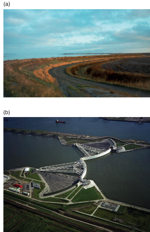
Figure 12.7 (a) Old sea defences fronting prime agricultural land at Wolfville, Nova Scotia. Photograph by David Pugh. (b) The Maaslantkering storm surge barrier in the Nieuwe Waterweg, Netherlands, which closes automatically when needed. Photograph from the Rijkswaterstaat, Dutch Ministry of Infrastructure and the Environment.
