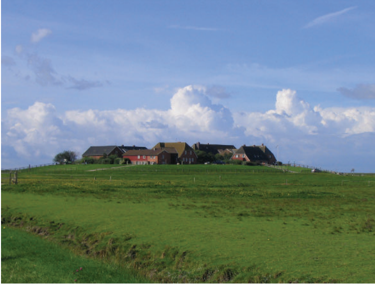
Figure 13.8 An artificial hill (terp) at Hooze in Germany, an example of many known to have been constructed in the coastal Netherlands, Germany and Denmark in approximately AD 0–1000. The terpen were mounds constructed to provide refuge during flooding. Photograph by Sandra Buhmann, a Wikimedia Commons image.43.
