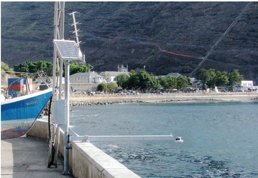
Figure 2.7 (a) A pair of acoustic tide gauges with satellite transmission on Easter Island. Photograph by David Pugh.
