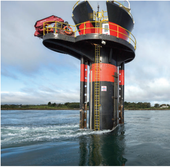
Figure 12.12 The 1.2 MW tidal stream generator at the entrance to Strangford Lough, Northern Ireland. Photograph supplied by Marine Current Turbines Ltd, a Siemens business.
