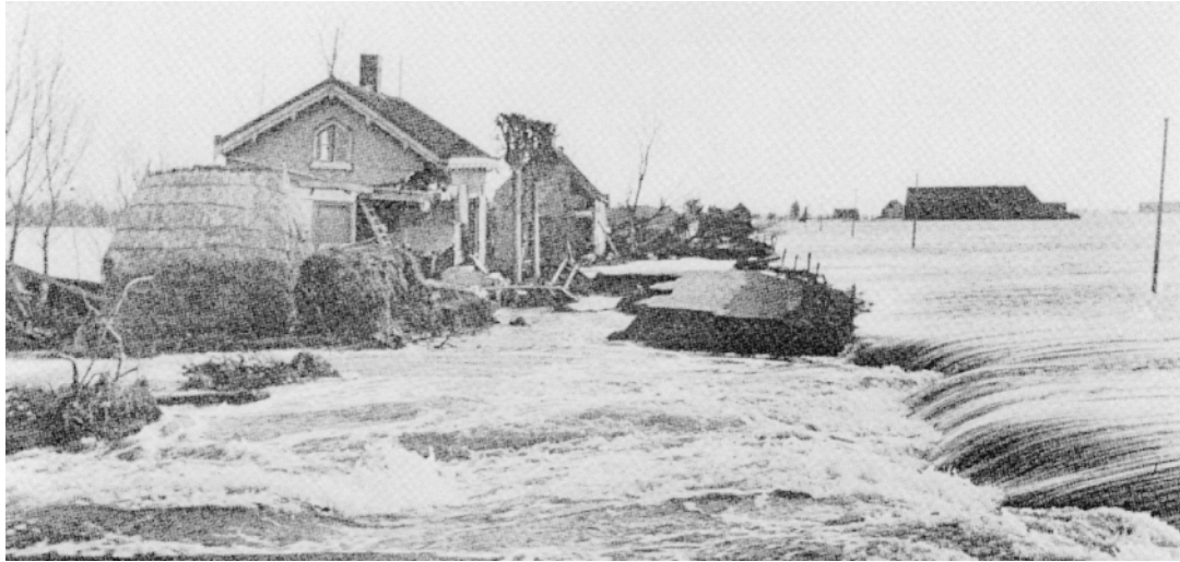
Figure 6 Breached dyke in the Netherlands after the 1953 North Sea storm surge. (Reproduced by permission of RIKZ, Ministry of Public Works, The Netherlands.)
