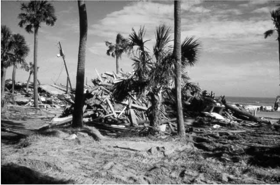
Figure 14.4 Damage to structure by Hurricane Opal in Florida.
