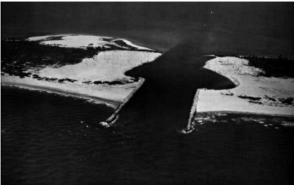
Figure 12.16 Inlet through St. George Island, Florida, showing wave-diffraction-induced channel bank erosion.
