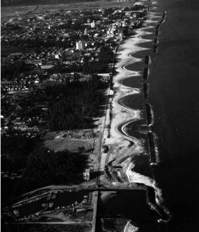
Figure 12.5 Multiple offshore breakwaters on the Kaike coast, Japan (courtesy of CTI Engineering Co., Ltd., and the Ministry of Construction, Chugoku Regional Construction Bureau, Hinogawa Work Office).
