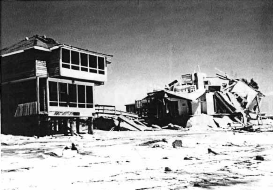
Figure 14.5 Damage to structure by Hurricane Hugo, Folly Island, South Carolina (Wang 1990).
