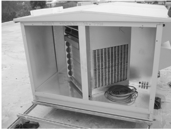
Figure 23.4 Air-to-air heat exchanger (Business Edge)
