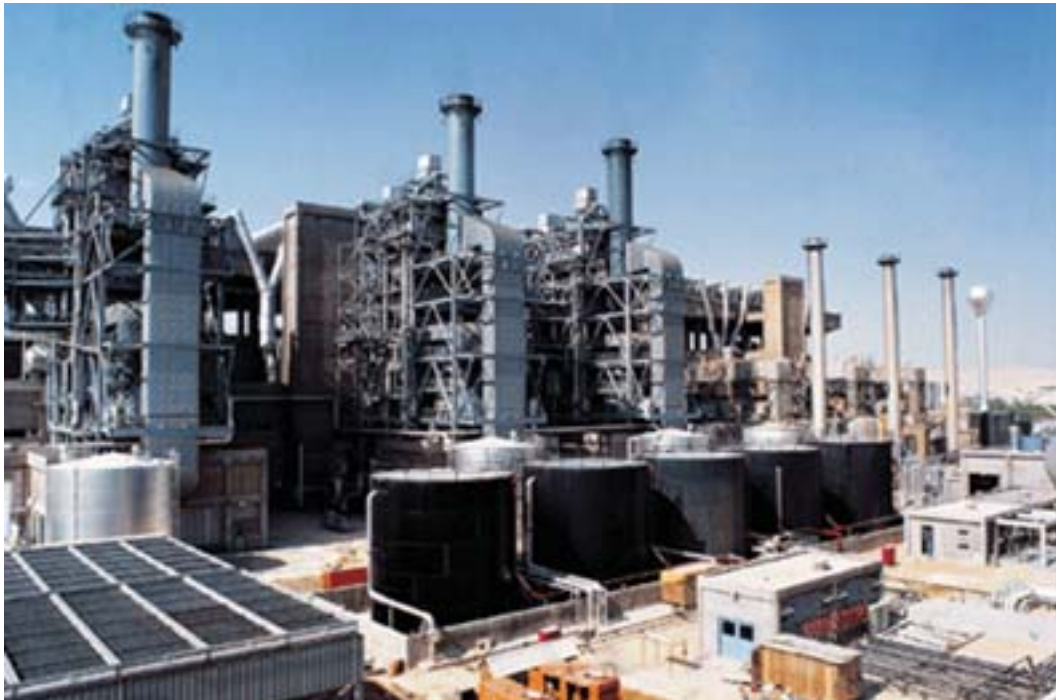
An overview of a thermal power station.
