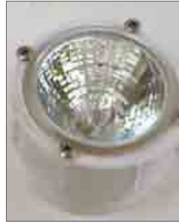
Retaining screws on a lamp.
