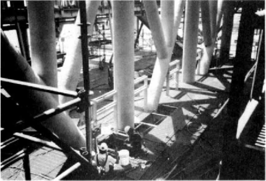
Fig. 9.30 Corrosion-resistant E-glass fiber-reinforced phenolic grating is 80% lighter than steel, has lower thermal conductivity, and meets strength and fire resistance requirements (courtesy MMFG).
