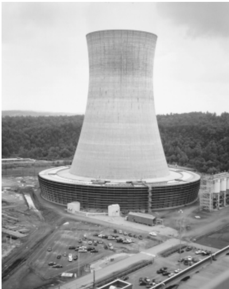
FIGURE 4.9.2 A natural-draft cross-flow cooling tower for a power plant.
