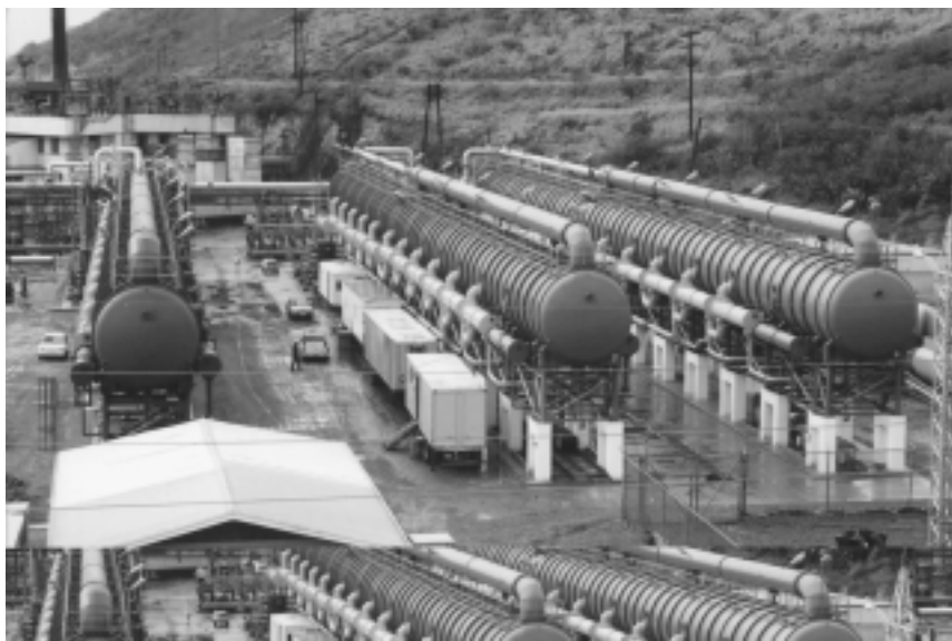
FIGURE 4.1.3 Two HTME desalination units, each producing 5000 m 3 /day, in St. Croix, U.S. Virgin Islands. (Courtesy of I.D.E. Technologies Ltd.)
