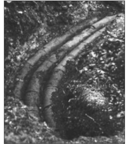
FIGURE 1–11 Segment of Pergamon pipeline. Each clay pipe section was 13 to 18 cm in diameter.
