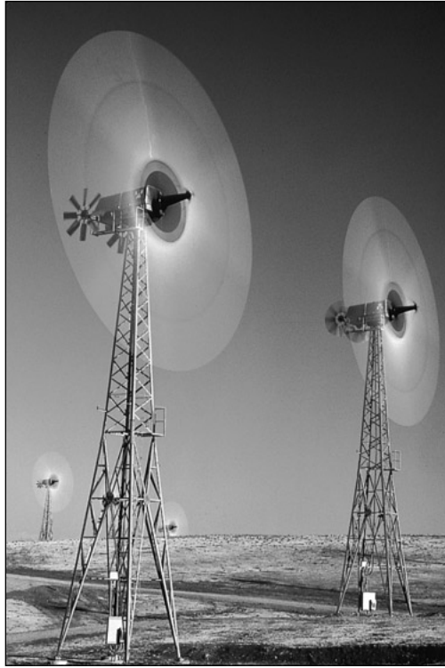
Wind-energy generator farm, Altamont Pass, California. Windmills have been used for power for more than two thousand years. These multi-bladed horizontal-axis wind turbines (HAWT's) are among the most efficient of windpower designs, as discussed in this chapter. (Courtesy of Kevin Schafer/Peter Arnold, Inc.)
