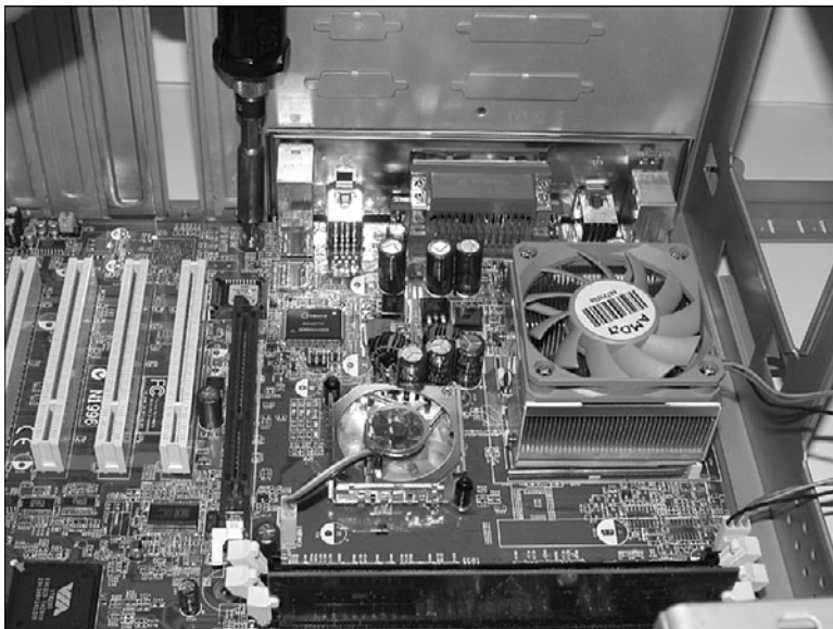
Figure 19.15 Installing the screws that hold the motherboard to the chassis.
