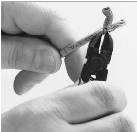
Figure 17.12 Carefully strip the cable jacket away to expose the four wire pairs.
