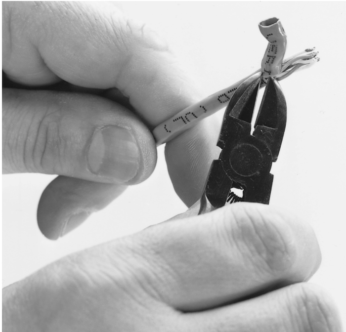
Figure 19.18 Carefully strip the cable jacket away to expose the four wire pairs.
