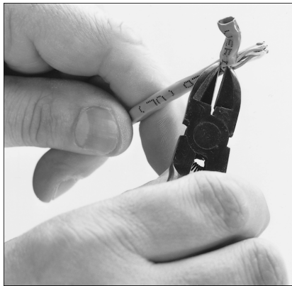
Figure 20.19 Carefully strip the cable jacket away to expose the four wire pairs.
