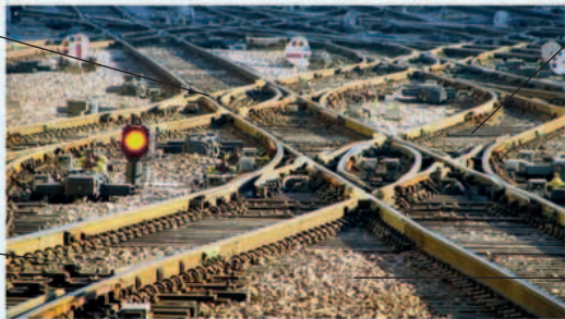
The rail is joined to ties, which keep the two rails the right distance apart.
