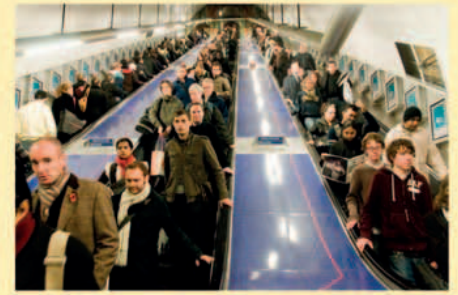
An escalator can carry more than 10,000 people in an hour.
