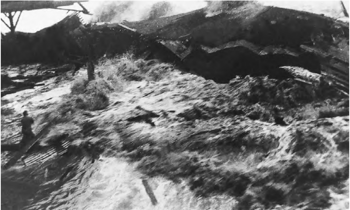
Tsunami inundating Hilo, Hawaii. National Oceanic and Atmospheric Administration (NOAA).
