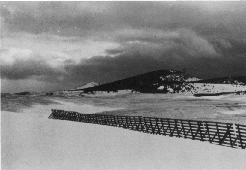
Fig. 1.8. Snow fence system (3.7 m high) along Interstate Highway 80 in Wyoming, USA. (Photograph by J. D. Iversen, 1979.)
