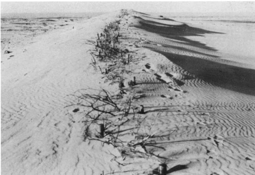
Fig. 1.9. Sand dune control in northern Denmark. Sand is trapped by a system of staggered poles and tree branches. (Photograph by J. D. Iversen, 1981.)
