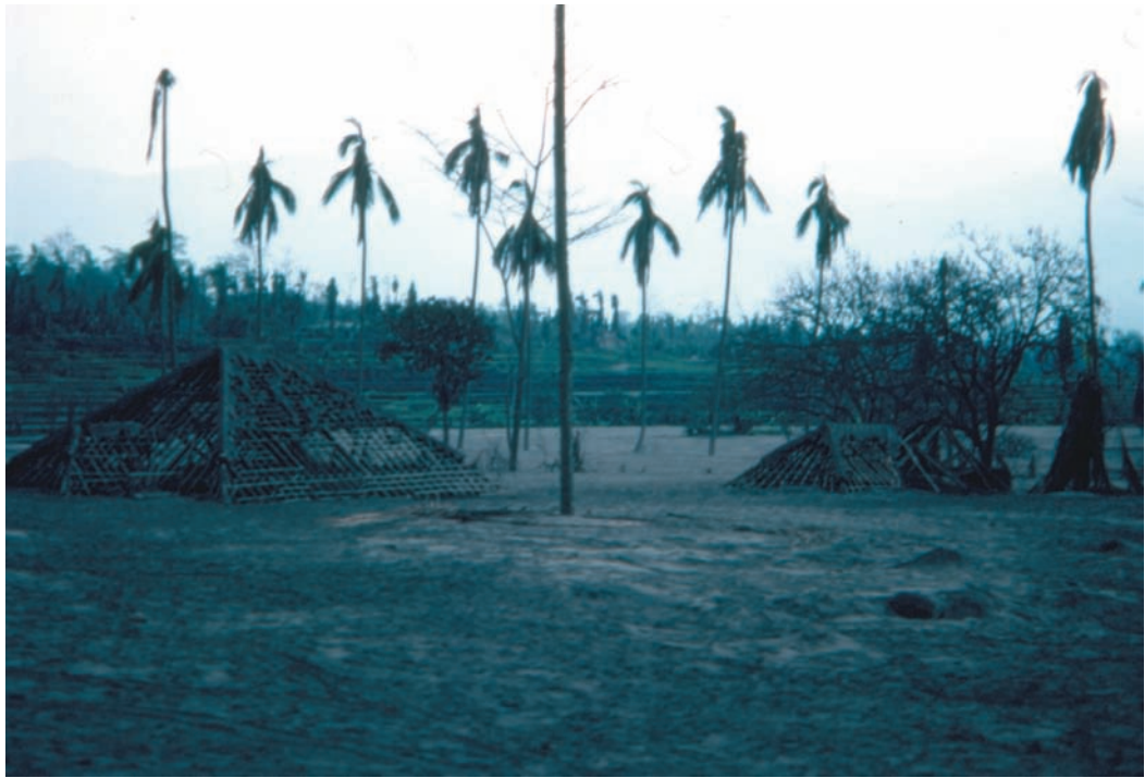
Fig. 11.14 Burial of homes in 1982 by hyperconcentrated flow deposits alongside Cibanjara River, 8 km below lahar sources, Galunggung volcano, Indonesia. Roof tiles have been salvaged from the abandoned homes. USGS photo by J. P. Lockwood.
