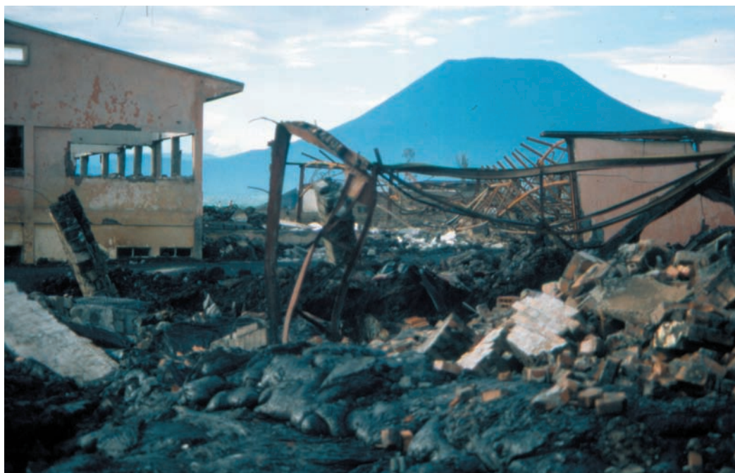
Fig. 14.2 View of Goma, eastern Democratic Republic of Congo, after fluid lavas poured through the city in 2002. Nyiragongo volcano, source of these lavas, looms over the city in the background. Highly fluid pāhoehoe lavas flowed around and through buildings, but ‘a`ā flows crushed any structures they encountered. Photo by J. P. Lockwood.
