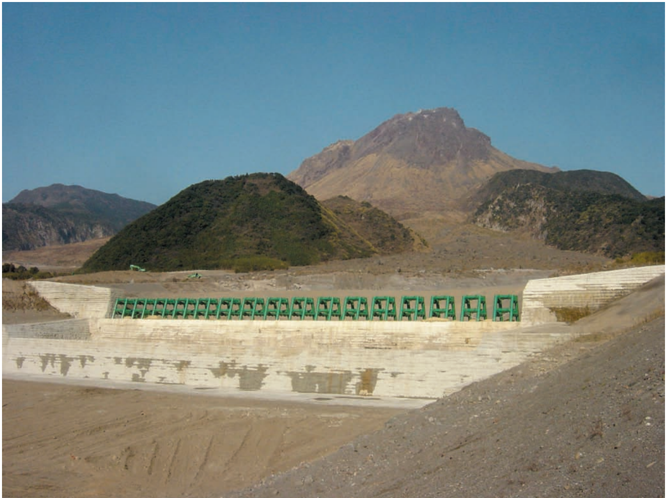
Fig. 14.17 Sabo dam for retarding lahars across the Mizunashi River system below Unzen [108] volcanic dome, Japan (in background). Dome growth in 1991 caused pyroclastic flows to move repeatedly down this river and set the stage for lahars and debris avalanches that remain a hazard at present. The sabo dam, 290 m wide and 10 m high, is designed to impound lahar deposits and to remove large lahar boulders by “filtering” them from lahars that may overtop the sabo. The lahar catchment basin above the sabo must be continuously excavated of debris to accommodate future lahar material. Photo courtesy of Etushi Sawada, Unzen Restoration Work Office, Nagasaki.
