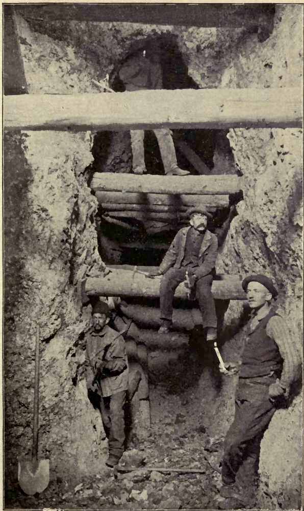
Down in a Gold Mine.
