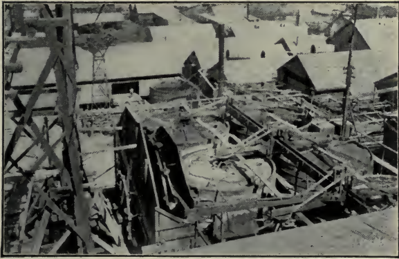
Cyanide plant, Lake View Consols.
