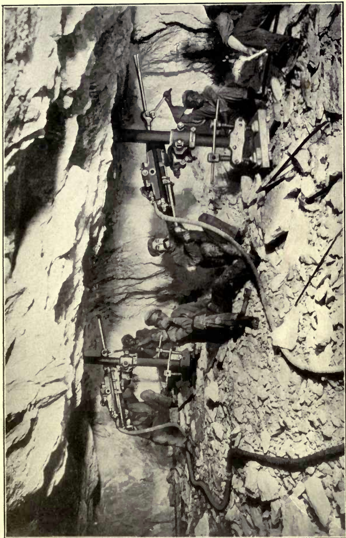
Drilling blast holes in a Rand Mine with Ingersoll Sergeant air-drills. The machines are fed through tubes from a steam compressor stationed above ground. These drills make upwards of 100 ft. holes in 10 min.
