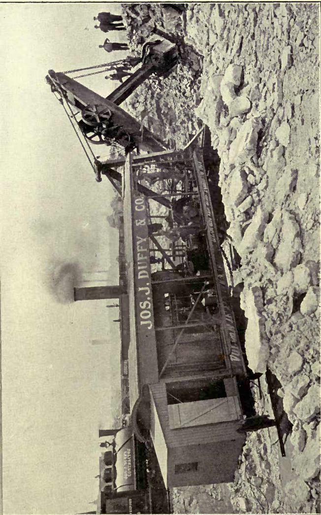
A Steam Shovel, such as is used in the Lake Superior iron-ore open-cast mines. The shovel raises five tons at each scoop, and will load a train at the rate of over ten tons a minute.
