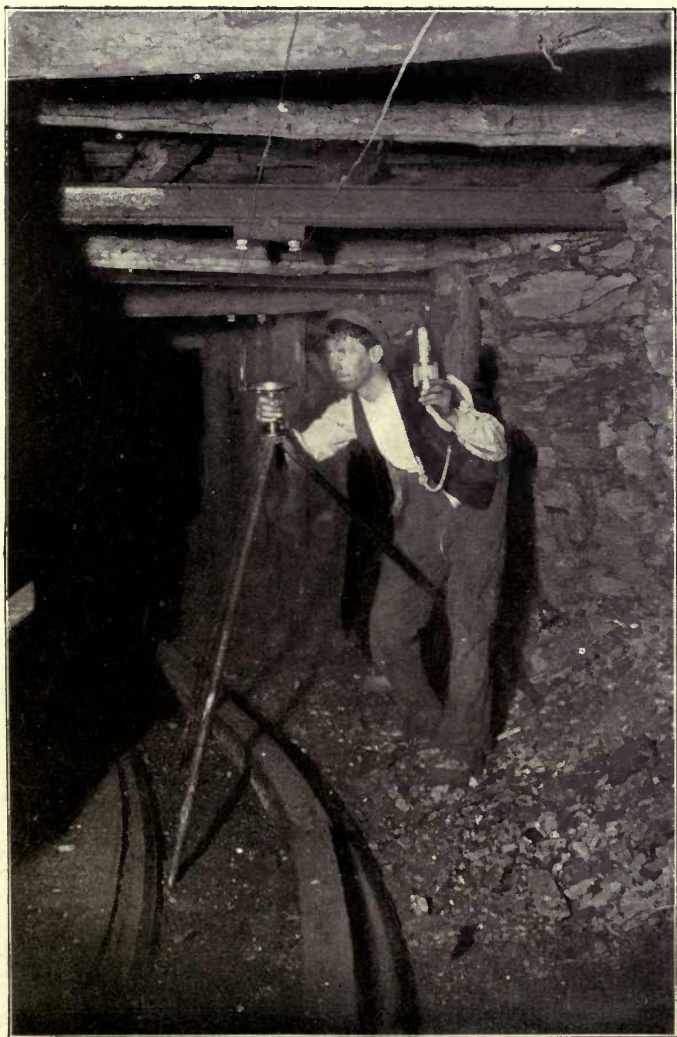
A mining surveyor at work in a coal mine. The position of every shaft, gallery, and heading in a mine is determined with great accuracy, and recorded on maps of the mine.
