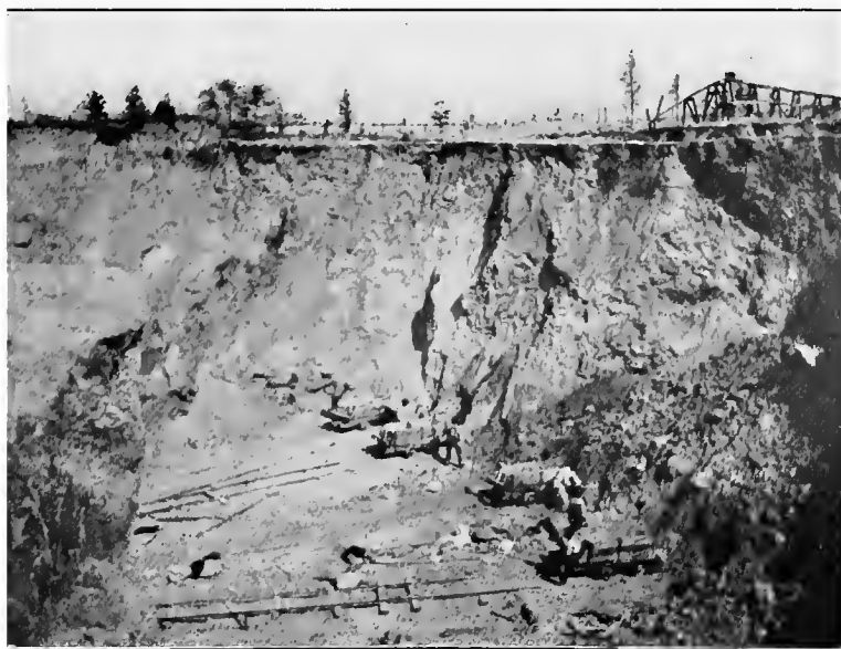
FIG. 2.—Phosphate Pit, Florida. [From a Photograph.] PLATE XXIV.
