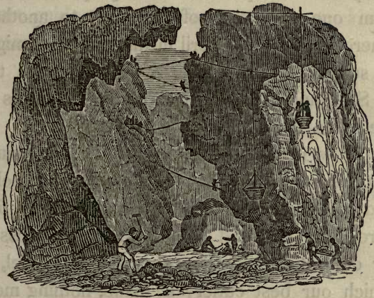
BORING THE ROCK FOR BLASTING.
