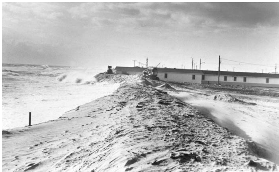
Figure 138 Serious losses of property near Cape Hatteras, Dare County, North Carolina, caused by shoreline regression and storm surges.
