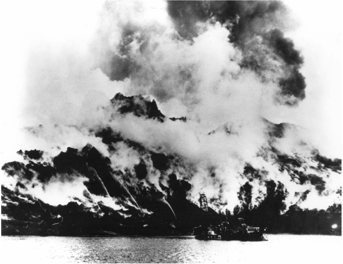
Figure 98 Seawater is sprayed onto the lava flow from the outer harbor of Vestmannaeyjar, Iceland, from the May 1973 eruption on Heimaey.
