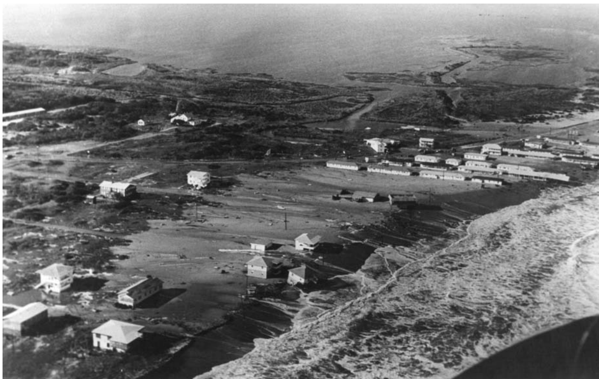
Figure 133 Overwash damage from storm surge at Cape Hatteras, North Carolina.
