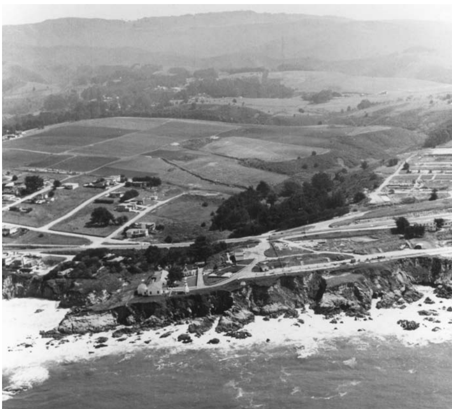
Figure 139 The erosion of these bluffs at Point Montara, California, will eventually deliver buildings, roads, and other structures to the sea.
