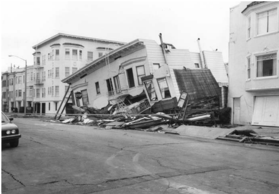
Figure 78 Collapsed buildings in the Marina District caused by the October 17, 1989, Loma Prieta earthquake, San Francisco, California.
