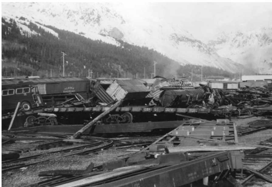
Figure 125 Seismic sea wave damage at railroad marshaling yard, Seward district, Alaska, from the March 27, 1964, earthquake.
