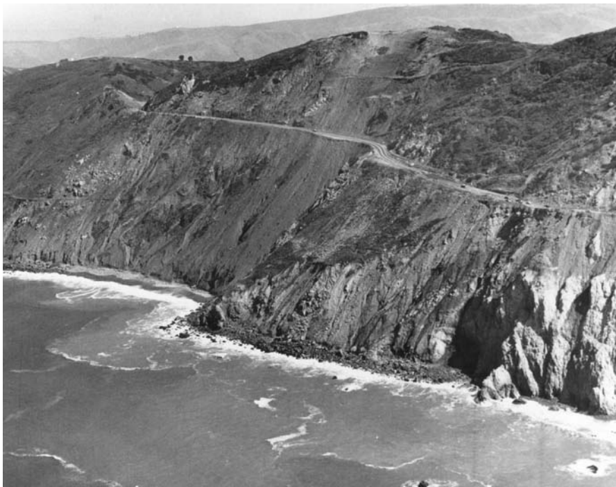
Figure 134 Highway 1 at the Devils Slide, San Mateo County, California.
