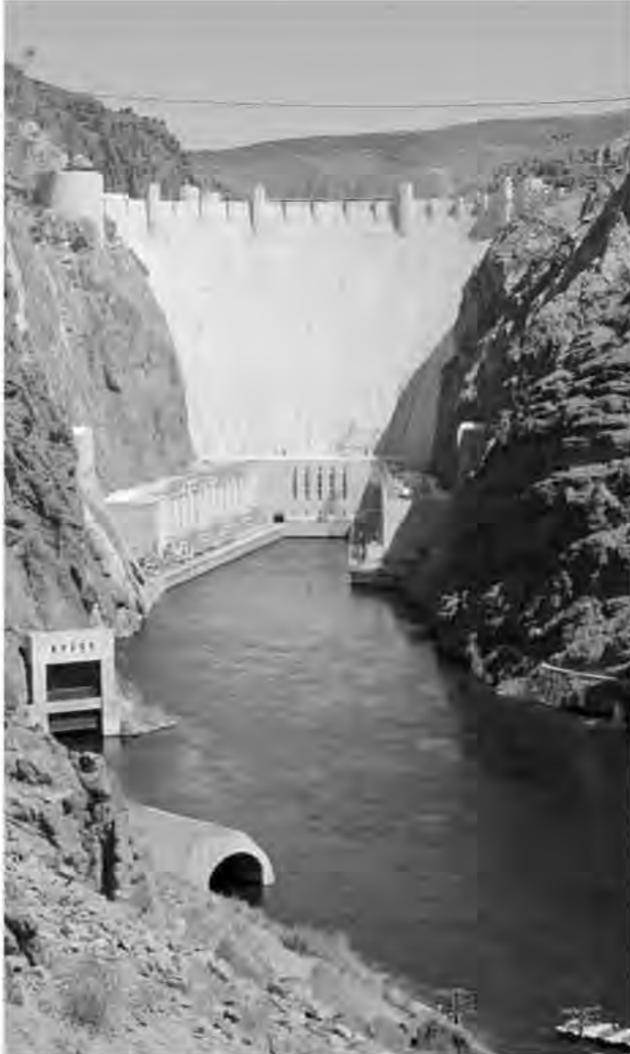
The giant Hoover Dam, the largest of the 50 dams controlling the 1,450-mile Colorado River, is shown near Boulder City, Nevada. AP/Wide World Photos.
