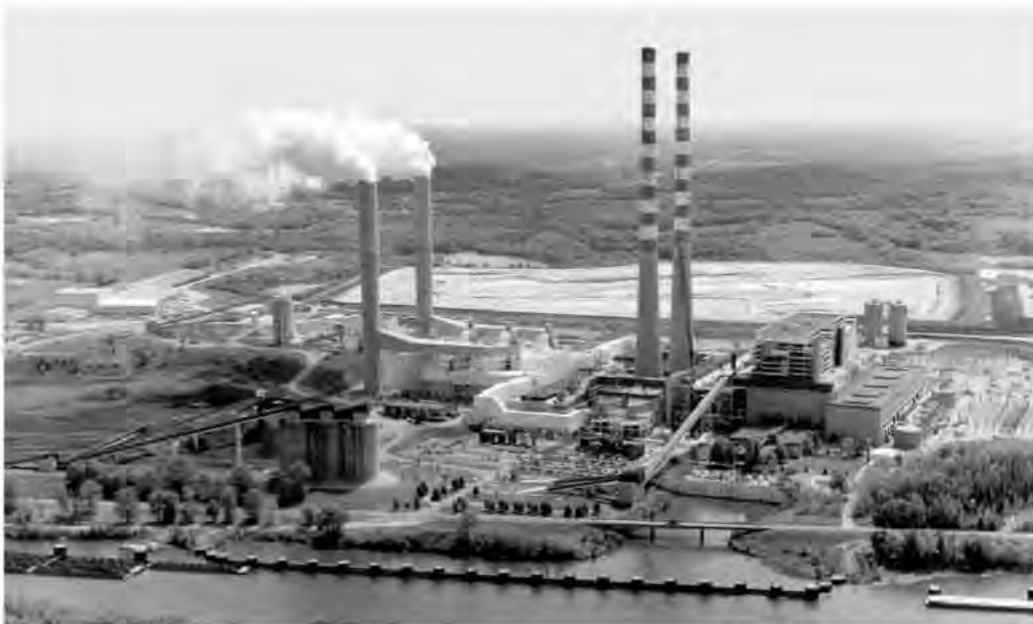
White plumes of water vapor rise from the two stacks of the emission scrubber system at the Tennessee Valley Authority's Cumberland Fossil Plant near Clarksville, Tennessee. The scrubbers reduce sulfur dioxide emissions that cause haze and acid rain. AP/Wide World Photos.
