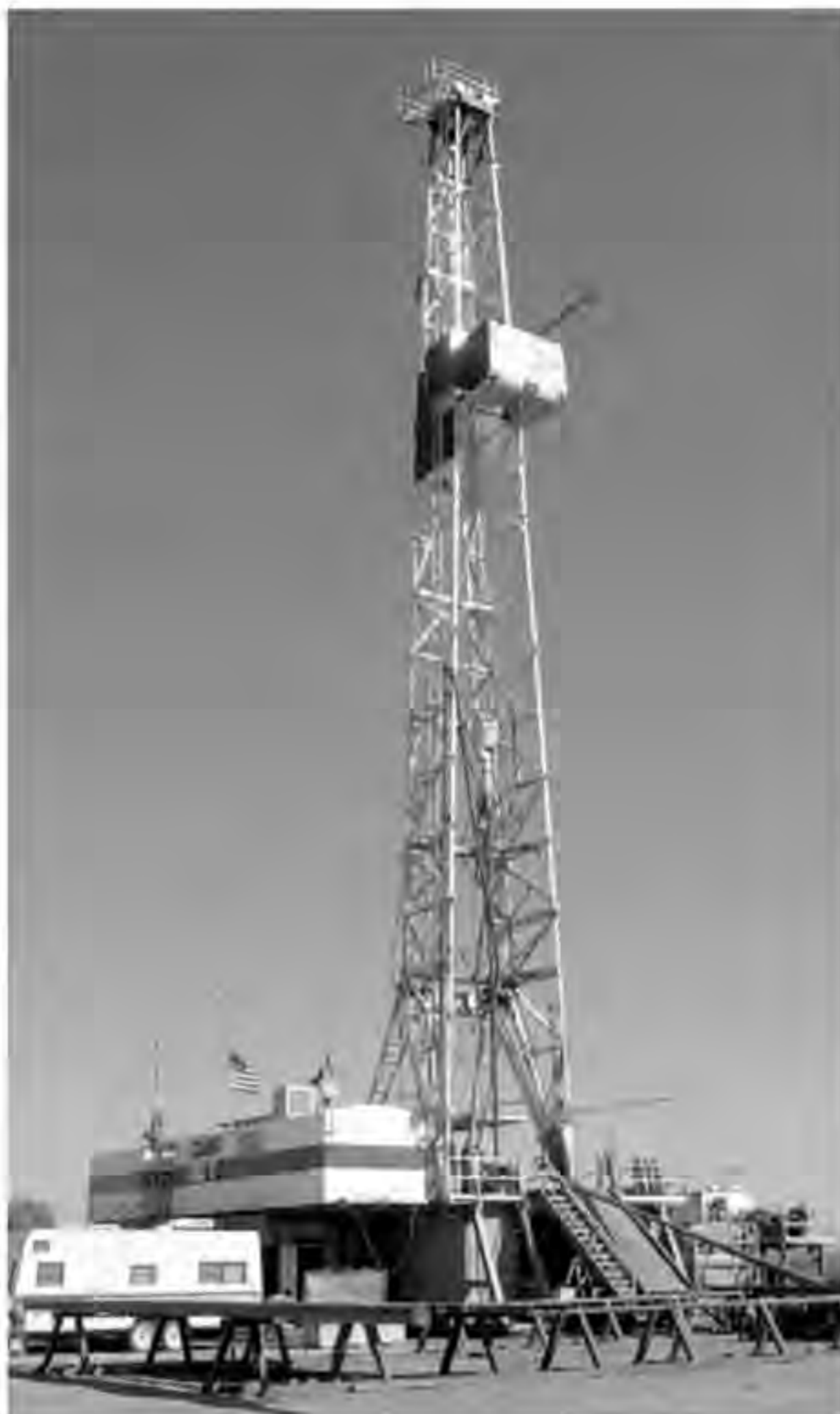
This oil drilling operation in Colorado features advanced drilling technology, resulting in thousands of gallons of water being saved and a reduction in truck traffic and waste. AP/Wide World Photos.
