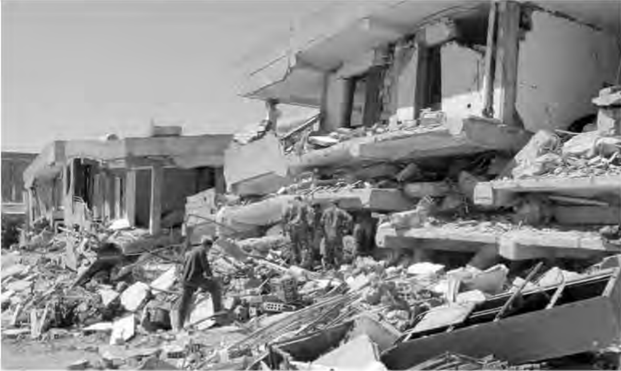
A man looks at the rubble of a building destroyed in Bumerdes, Algeria, after an earthquake struck the region on May 21, 2003. It was estimated that more than 1,500 people died and more than 7,200 people were injured in this quake, which registered 6.7 on the open-ended Richter scale. AP/Wide World Photos.
