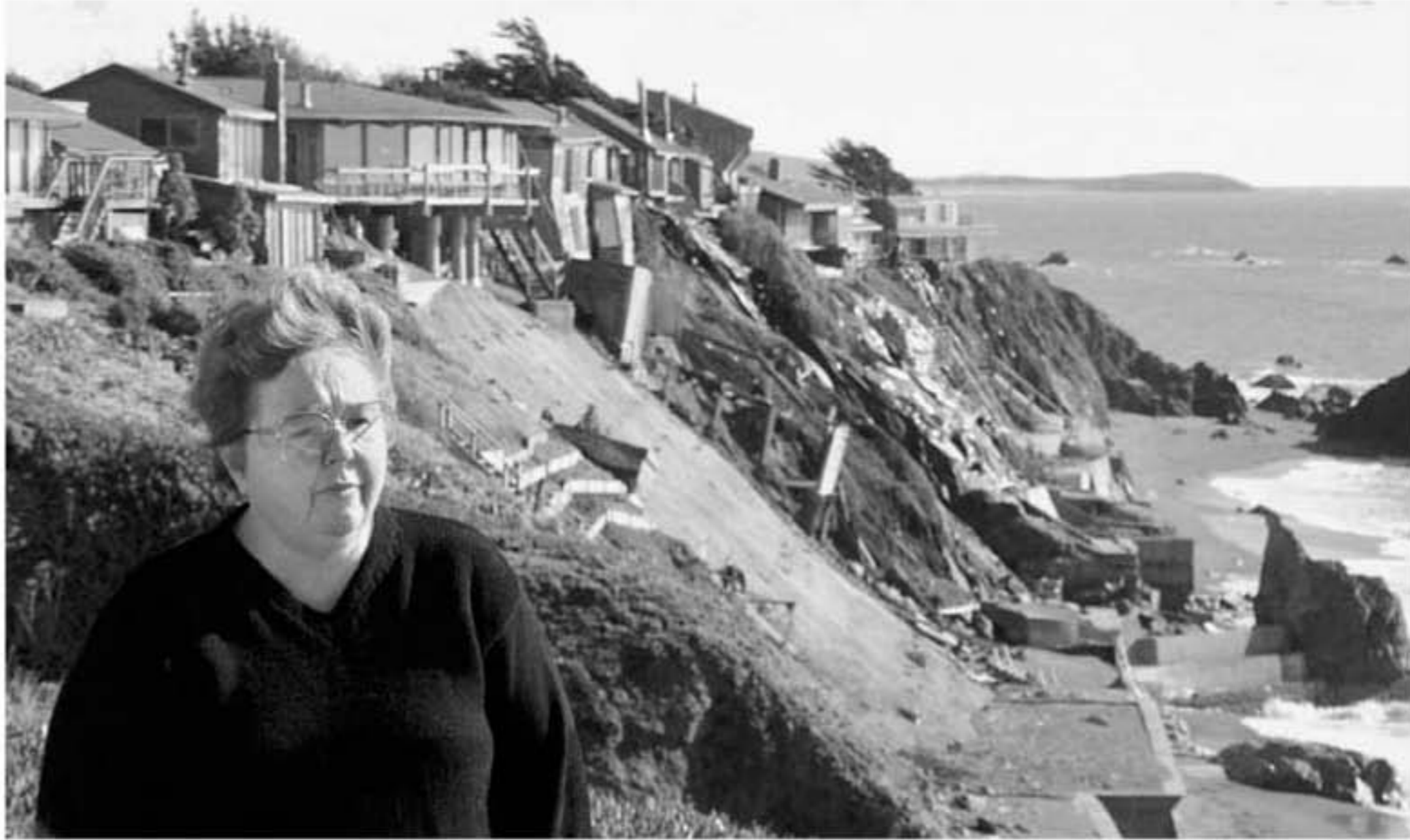
A resident stands in front of her oceanfront house in Bodega Bay, California, where El Niño-driven storms eroded the cliffs below, threatening to send her house and several others plunging into the Pacific Ocean. AP/Wide World Photos.
