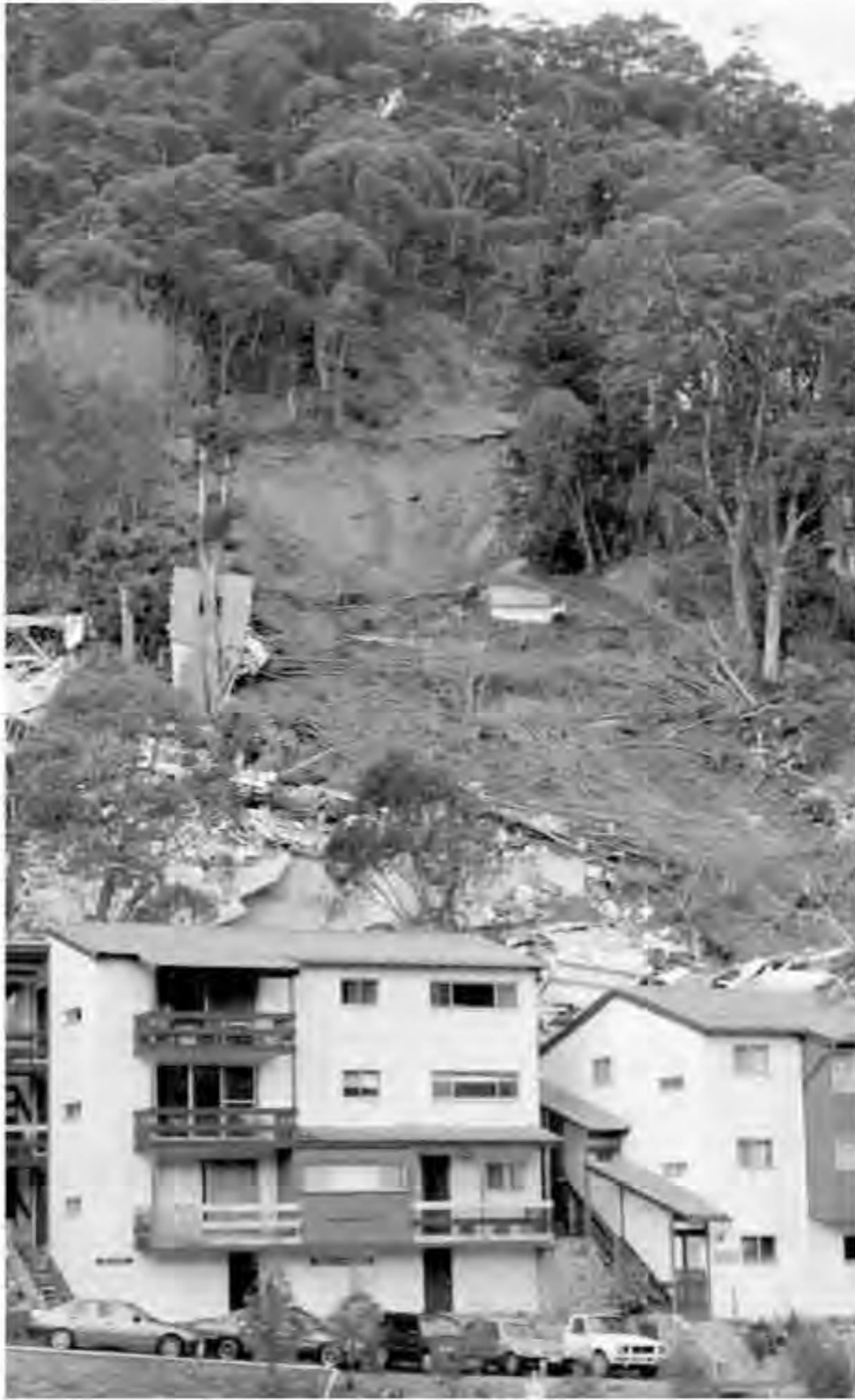
An aerial view of the landslide and remains of flattened ski lodges at the Australian resort of Thredbo taken July 31, 1997. Landslides occur all over the world, and in the United States, cause almost $2 billion in damages yearly. AP/Wide World Photos.
