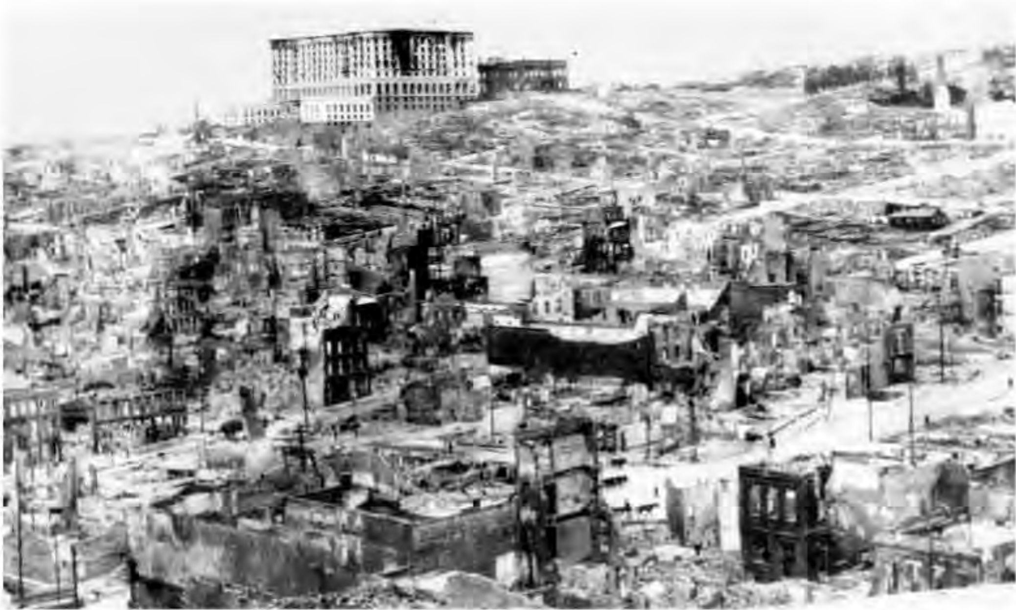
A view of the destruction resulting from the April 18, 1906, earthquake in San Francisco, California. Following the powerful quake, fire spread throughout the city reducing much of the remaining structures to rubble. AP/Wide World Photos.
