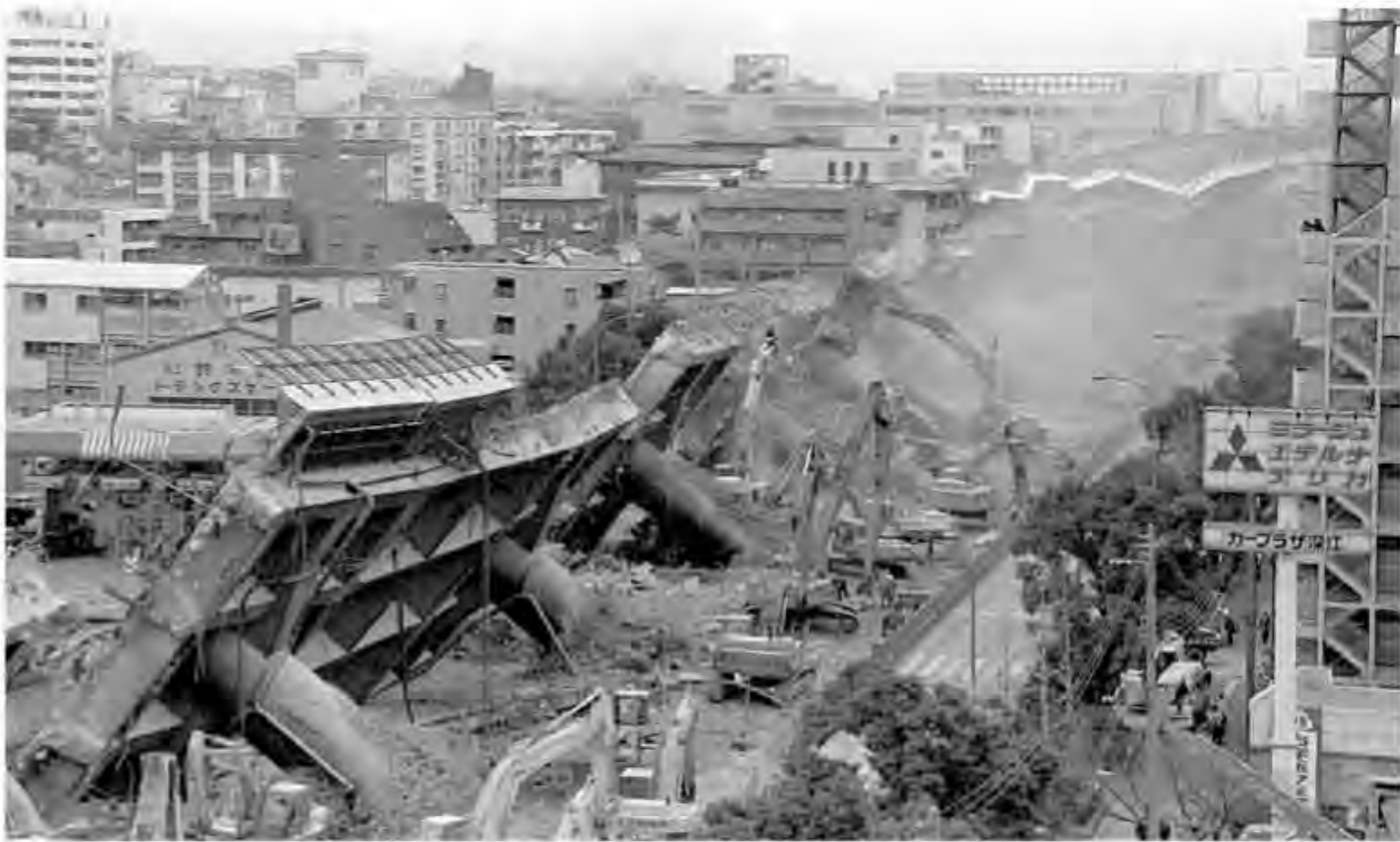
Heavy construction machines break up concrete from a toppled freeway in Kobe, Japan. Portions of the Kobe-Osaka freeway collapsed during the earthquake that hit this western Japanese city early on January 17, 1995. AP/Wide World Photos.
