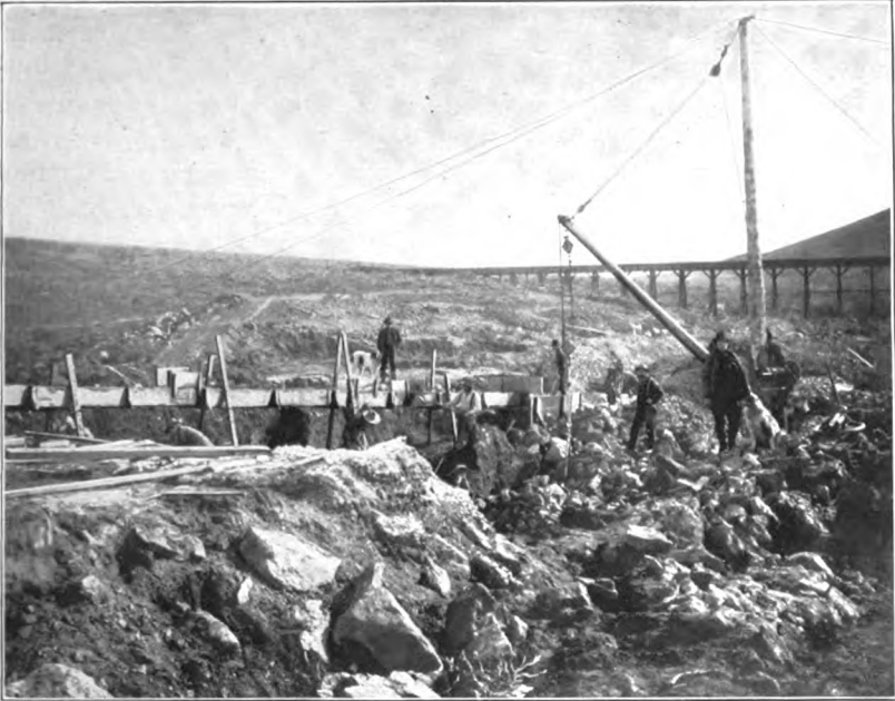
A. ROUGH BOWLERS IN THE PAY STREAK OF A PLACER MINE ON CROOKED CREEK.
