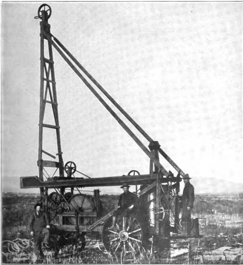
B. PROSPECTING FOR PLACER GOLD WITH CHURN DRILL NEAR BLUFF.
