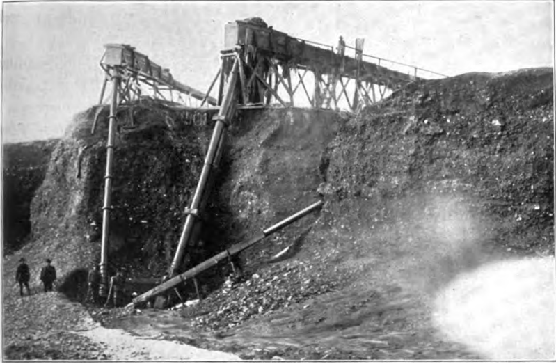
A. HYDRAULIC ELEVATOR ON GLACIER CREEK.
