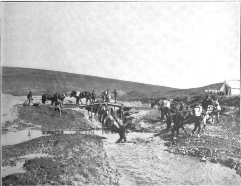
B. MINING WITH HORSES AND SCRAPERS ON GOLDBOTTOM CREEK.
