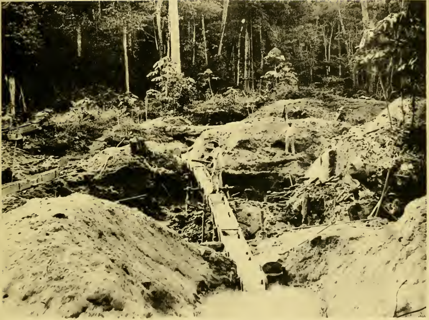
PLACER WORKING. SLUICE AND TAILINGS.
