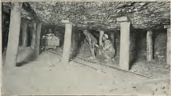
FIG. 117.—Prop and lid, alluvial gold mine, Western Australia.
