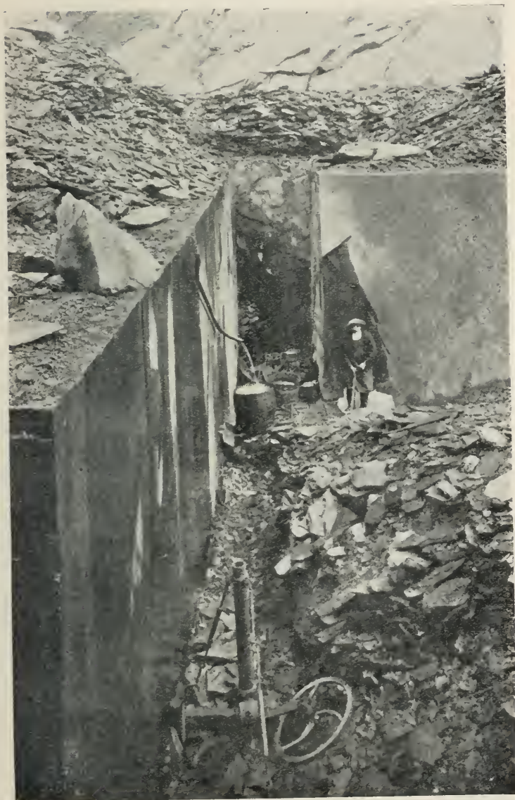
FIG. 93.—Maillou Slate Quarry, Labassère, near Bagnères-de-Bigorre, France, where vertical and horizontal cuts are made by the wire-saw. The horizontal cuts in the picture are covered by rubbish.*
