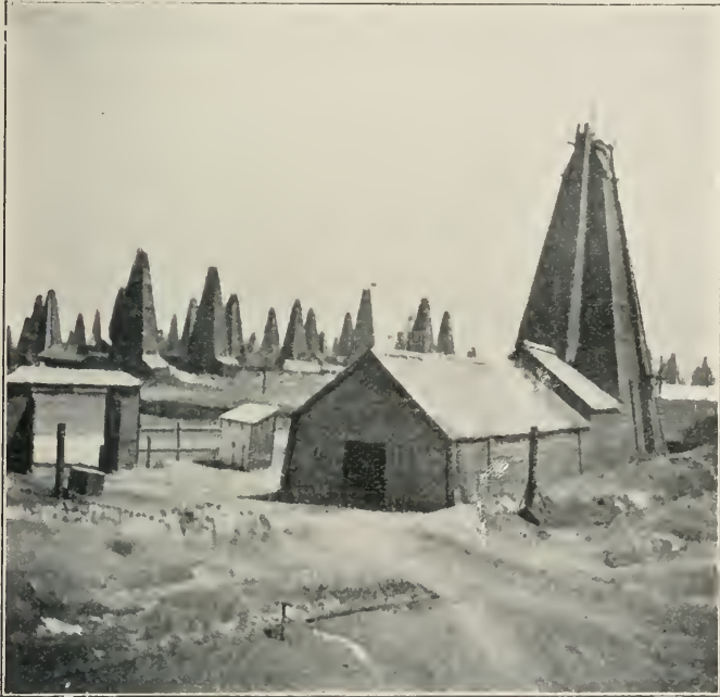
FIG. 145.—A small portion of the Balakhany oil-field, near Baku, Russia, with numerous derricks, each one over a borehole.
