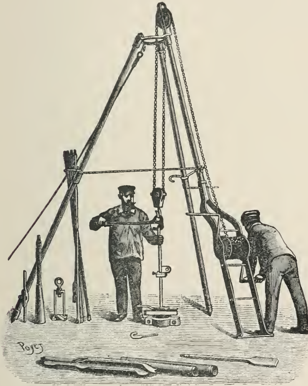
FIG. 33.—Arrault's small portable Boring Plant.
