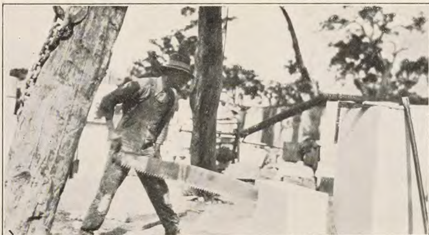
Sawing Polyzoal Limestone into Building Blocks, near Mount Gambier.
