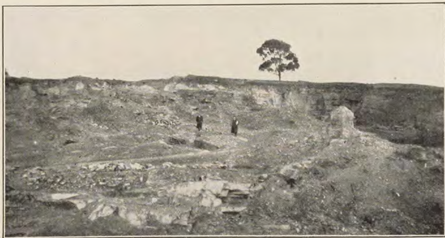
Tarlee Slate Quarry, Section 215, Hundred of Gilbert.
