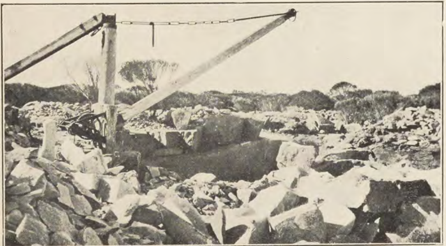
Monarto Granite Quarry, Section 520, Hundred of Mobilong.
