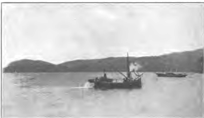
The salvage steamer Breamer equipped with suction dredge, removing a sandbank from the supposed location of the Florencia galleon in 1909.
