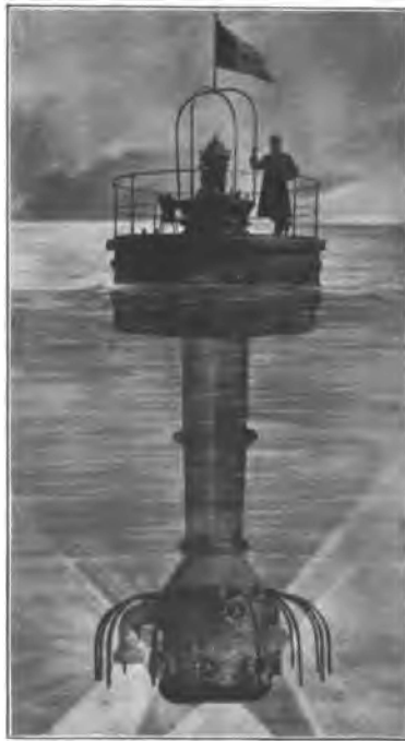
Hydroscope invented by Pino for exploring the sea bottom and successfully used in finding the galleons of Vigo Bay. (By permission of The World's Work, London.)
