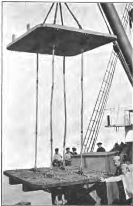
Framework of an "elevator" devised by Pino for raising the galleons in Vigo Bay.
