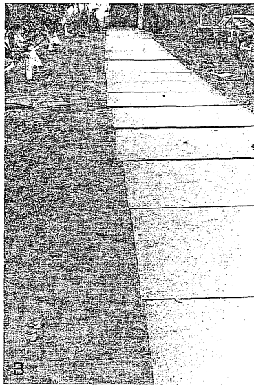
Figure 2.15 (A) Schematic portrayal of horizontal, left-handed slip on a vertical fault. The magnitude of translation is 5 cm. (B) Real-life examples of horizontal, left-handed slip on vertical faults. The sidewalk panels were shifted by faulting during the earthquake in Managua, Nicaragua, in 1972. Faulting of the sidewalk took advantage of preexisting discontinuities. Maximum translation is about 3 cm. Aggregate displacement across the 12-m wide exposed zone is 28.6 cm. (Photograph by R. D. Brown, Jr. Courtesy of United States Geological Survey.)
