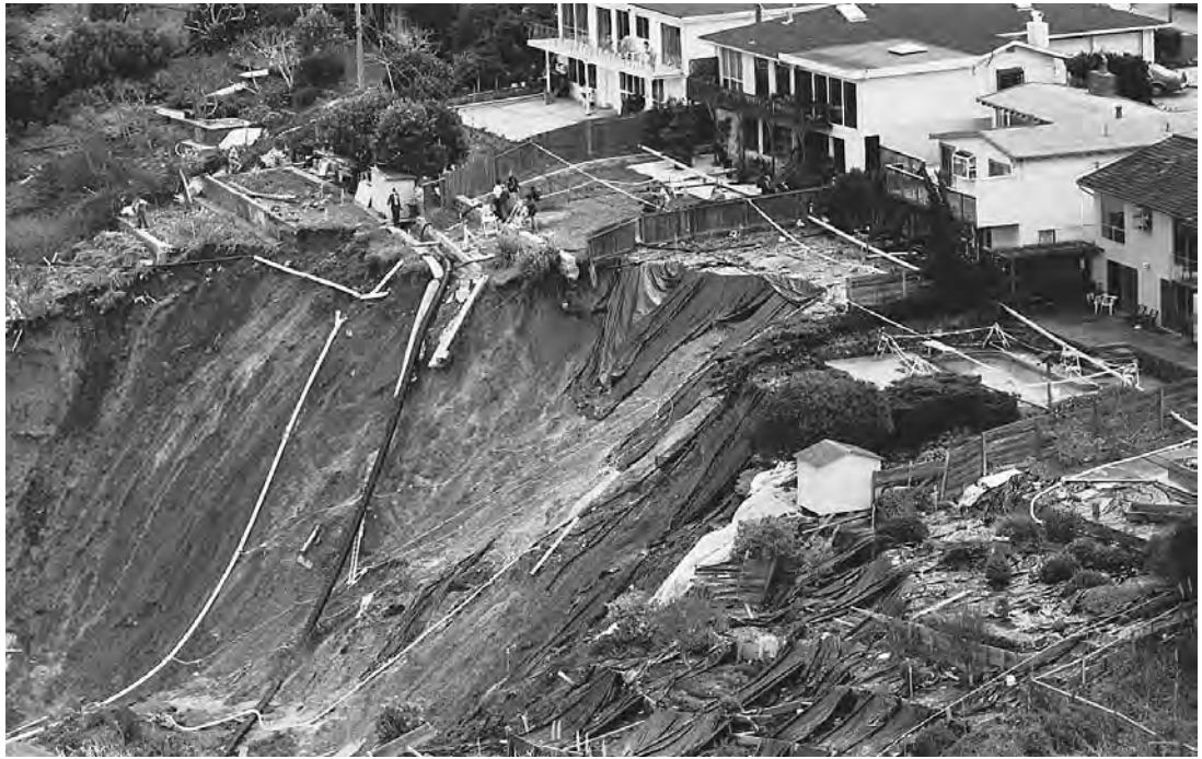
A MUDFLOW CAUSED BY HEAVY WINTER RAINS BRINGS DOWN THE HILLSIDE UNDER HOMES IN MILLBRAE, CALIFORNIA. (AP/Wide World Photos. Reproduced by permission.)
