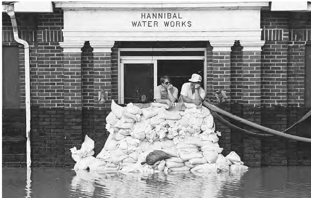
THE FLOODWATERS OF THE MISSISSIPPI RISE TO 4 FT. (1.2 M), SURROUNDING THE PUMPING STATION IN HANNIBAL, MISSOURI. APART FROM NATURAL CAUSES, FLOODS CAN RESULT FROM INCONSISTENT FLOOD MANAGEMENT, POOR CIVIL ENGINEERING DESIGN, AND UNWISE AGRICULTURAL PRACTICES. (AP/Wide World Photos. Reproduced by permission.)
