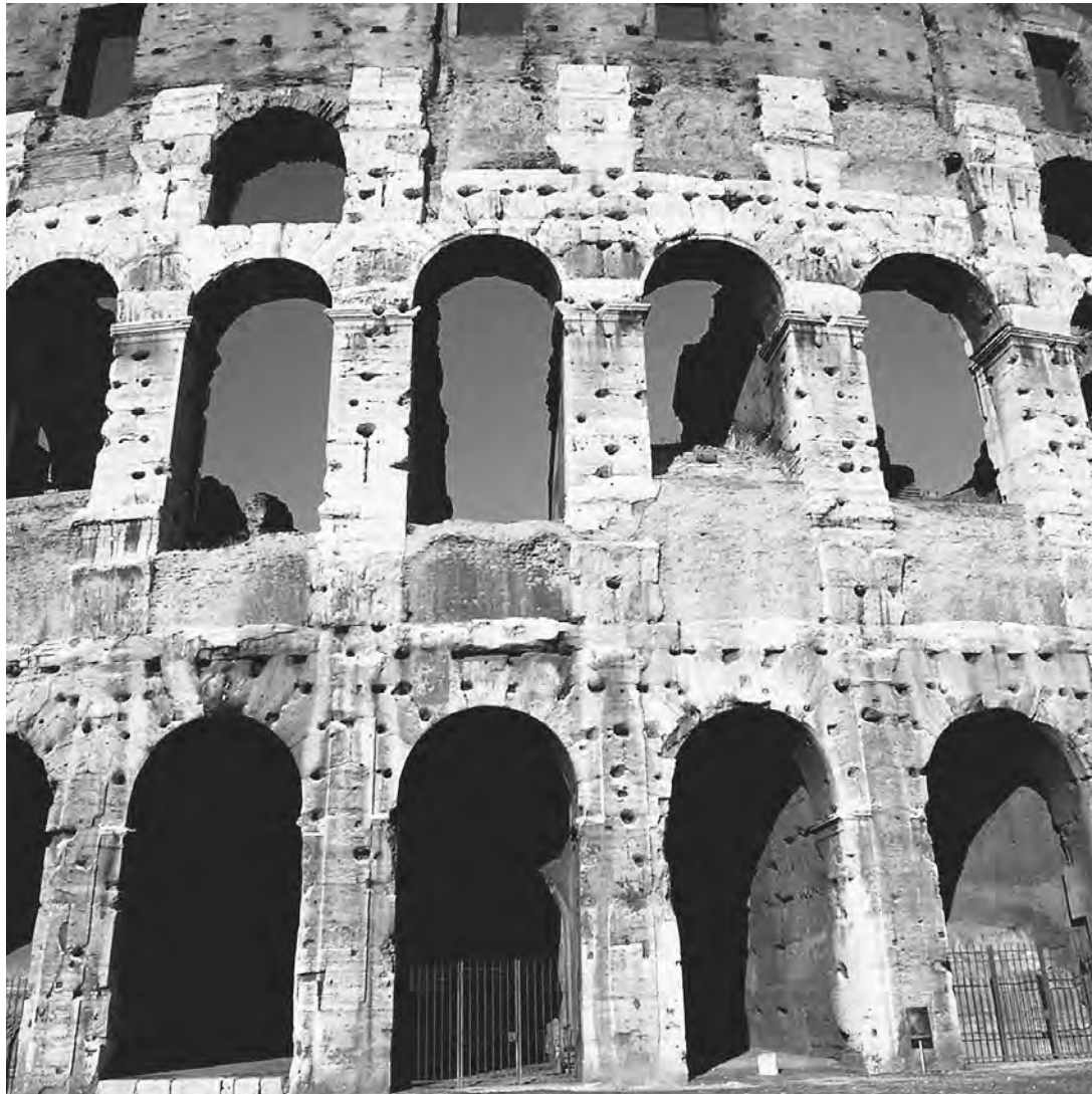
WHILE STONE IS A STRONG BUILDING MATERIAL IN TERMS OF COMPRESSION, IT IS WEAK IN TERMS OF TENSION. THE ARCH OWES ITS STRENGTH TO THE PRINCIPLE OF WEIGHT DISTRIBUTION, WHICH OVERCOMES THIS SHORTCOMING OF STONE. INDEED, THE ROMAN COLISEUM HAS STOOD FOR MORE THAN TWO THOUSAND YEARS. (© John Moss/Photo Researchers. Reproduced by permission.)
