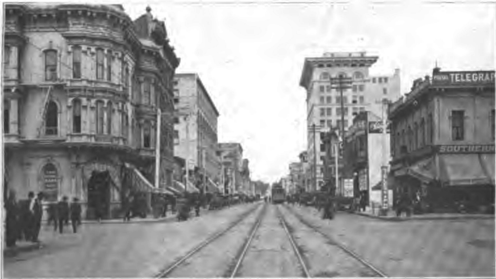
FIFTH STREET, LOOKING NORTH FROM E STREET
