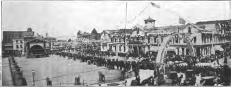
HORTON HOUSE AND PLAZA IN 1899 Present Site of U. S. Grant Hotel
