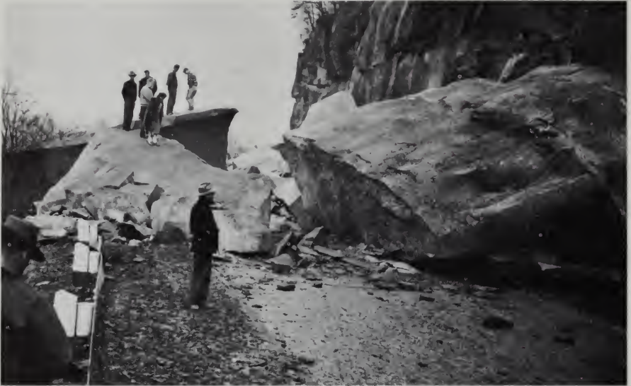
FIG. 22.8. Rockfall on State Route 7, Washington County, Ohio. (Photo by Ohio Department of Highways.)
