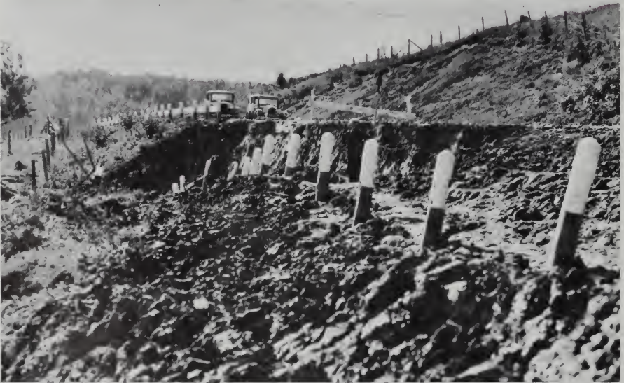
FIG. 22.9. Slumping of a road built upon plastic lacustrine material, Bayfield County, Wisconsin. (Photo by Wisconsin Geol. Survey.)
