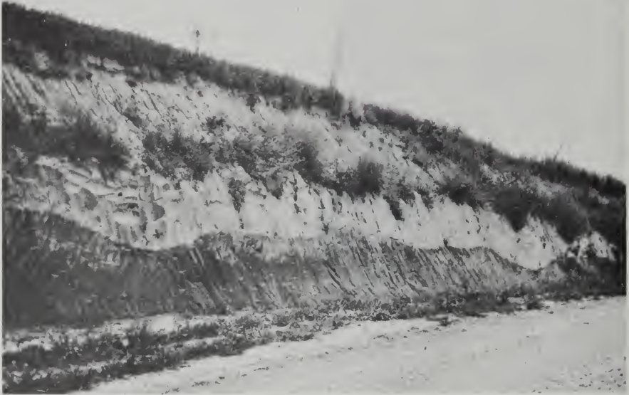
FIG. 16.18. A roadcut through loess showing the line of contact between leached and unleached loess. This can rarely be seen. Special circumstances are responsible for its showing so well in this picture.
