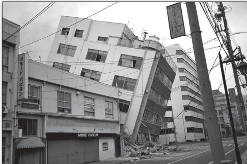
Building knocked off its foundation by the January 1995 earthquake in Kōbe, Japan. Dr. Roger Hutchison/NGDC
