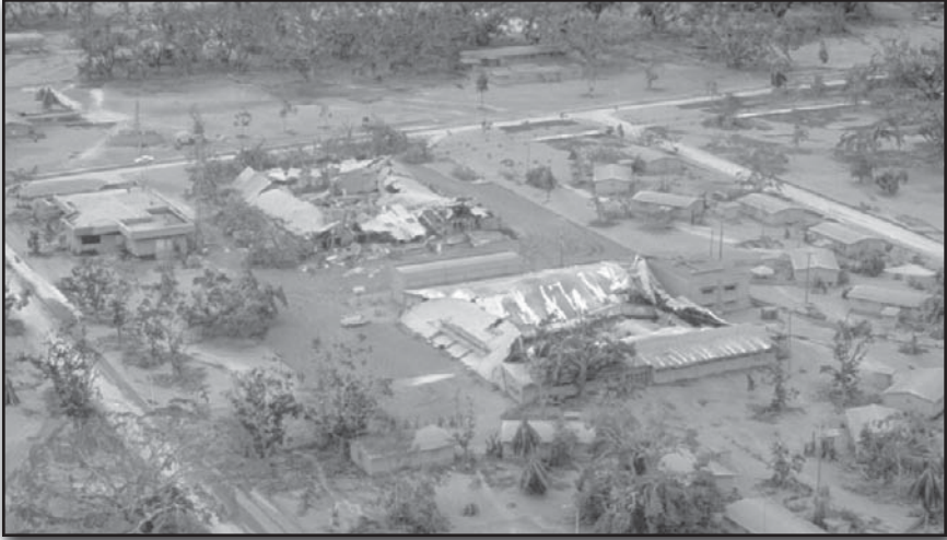
Buildings and vegetation at Clark Air Base, Philippines, are destroyed by a thick, wet layer of ash following the gigantic explosion of Mount Pinatubo on June 15, 1991. Willie Scott/U.S. Geological Survey
