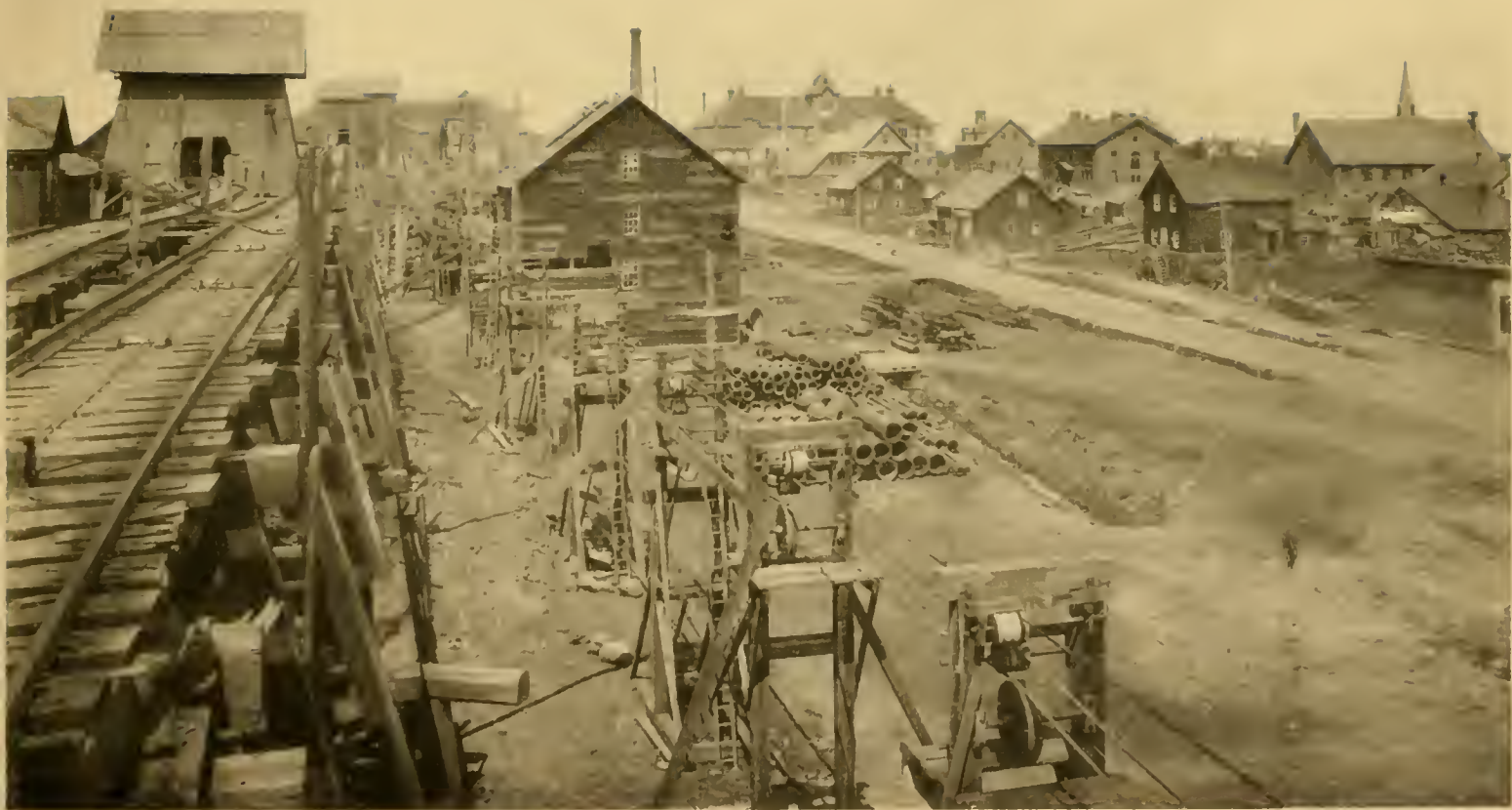
CALUMET, LOOKING EAST FROM SHAFT 2
