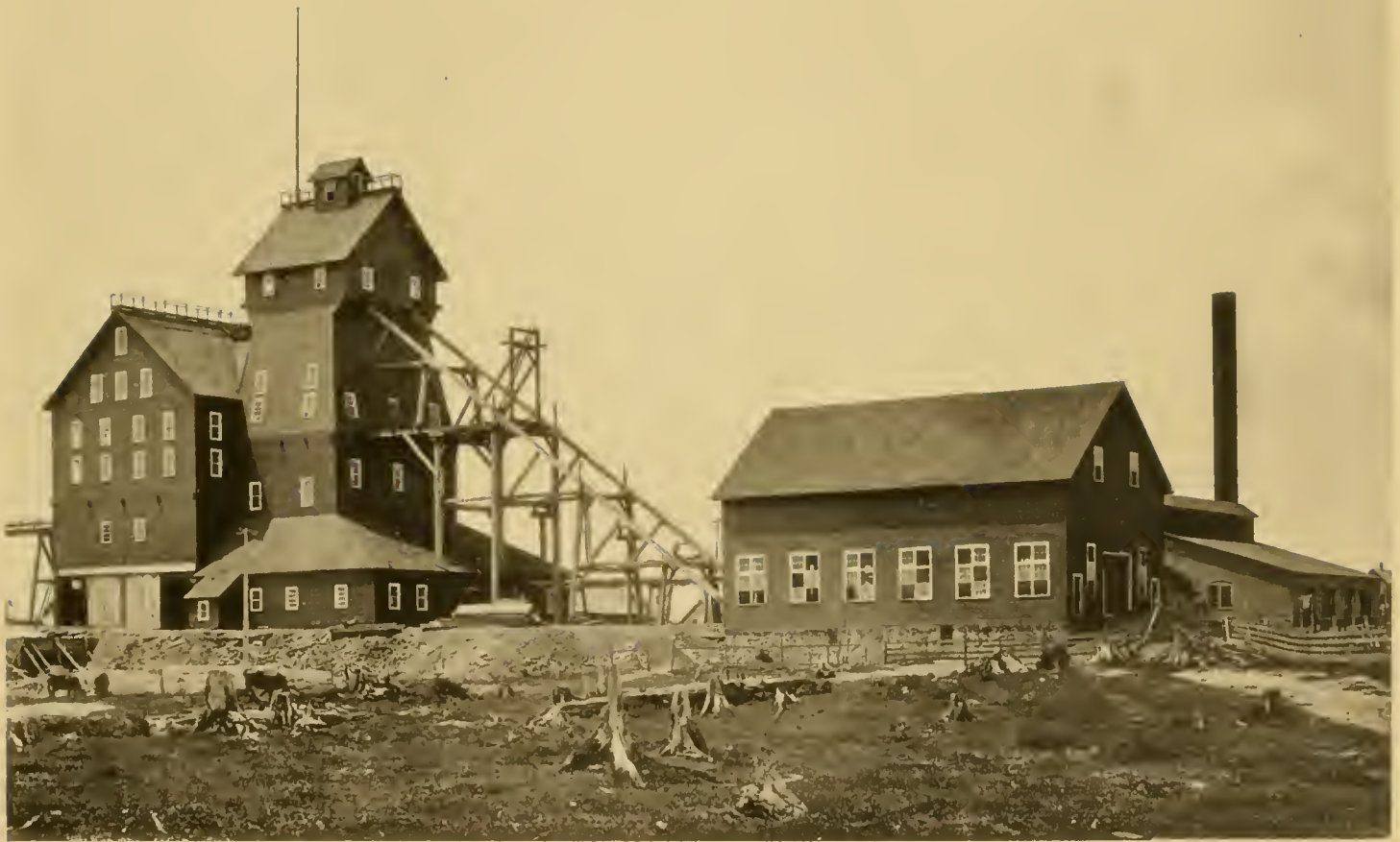
TAMERICK MINE ROCK AND SHAFT HOUSE.
