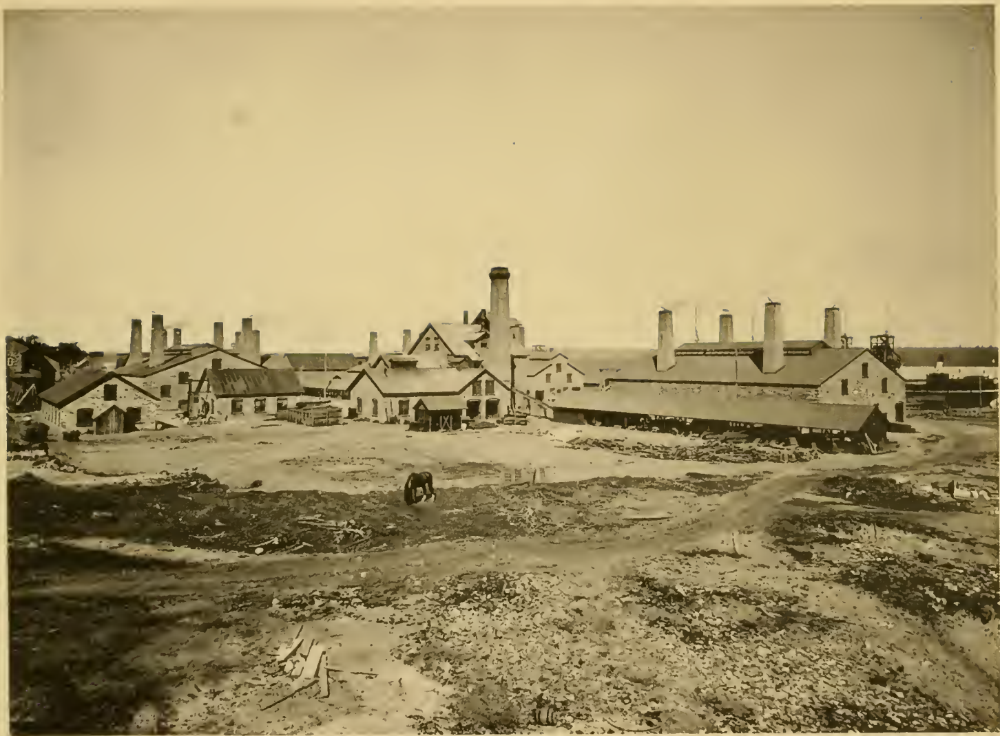
GRONE'S SMELTING WORKS SOUTH LAKE LINDEN
