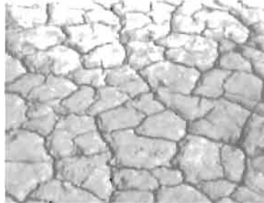
c) Crack network observed in mud.
