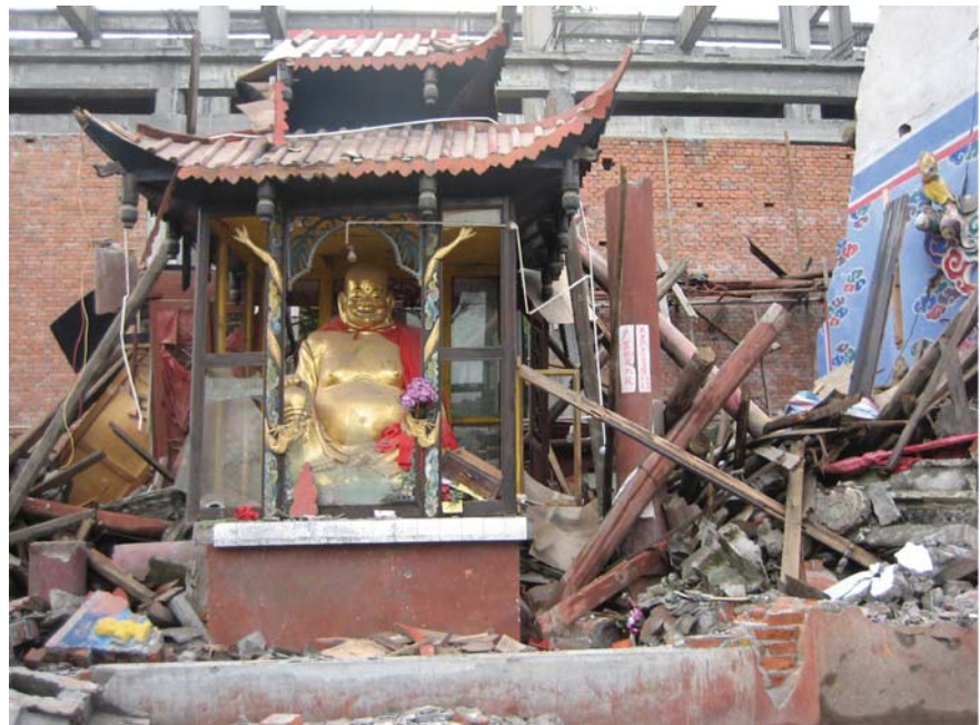
Fig. 16 Ruins of an ancient temple in Hanwang-Mianzhu, Sichuan, China. The destruction of the Wenchuan, China, earthquake reinforces the point that a long recurrence interval is not equivalent to safety. This temple withstood hundreds of years of environmental forces but was destroyed by the M_w = 7.9 earthquake on May 12, 2008. Source: Sarah Bahan, USGS
