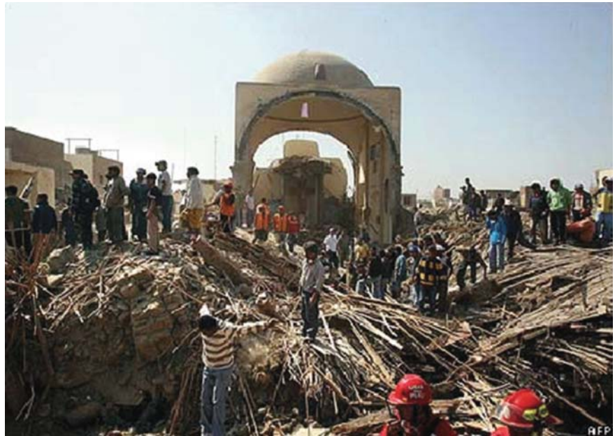
Fig. 10 Rescue workers and local residents search for survivors in the rubble following the August 15, 2007, M_w = 8.0 Pisco, Peru earthquake. Many of the deaths and injuries occurred in homes constructed with highly vulnerable adobe bricks
