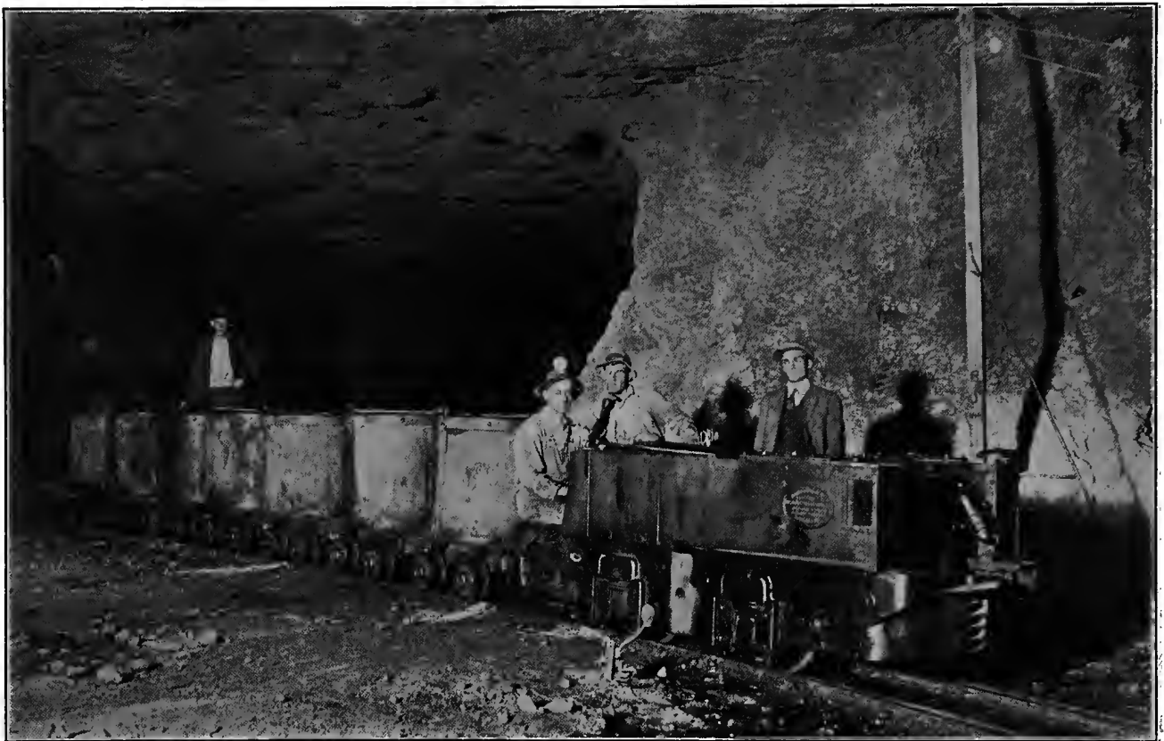
FIG. 9. UNDERGROUND HAULAGE IN THE JOPLIN DISTRICT WITH STORAGE-BATTERY LOCOMOTIVE
