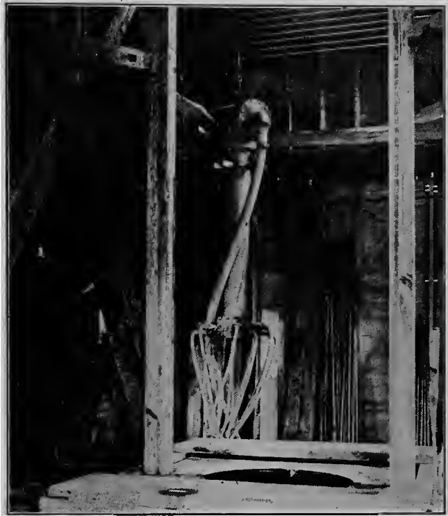
AIR HEADER USED IN SINKING SENECA SHAFT, MOHAWK, MICHIGAN
