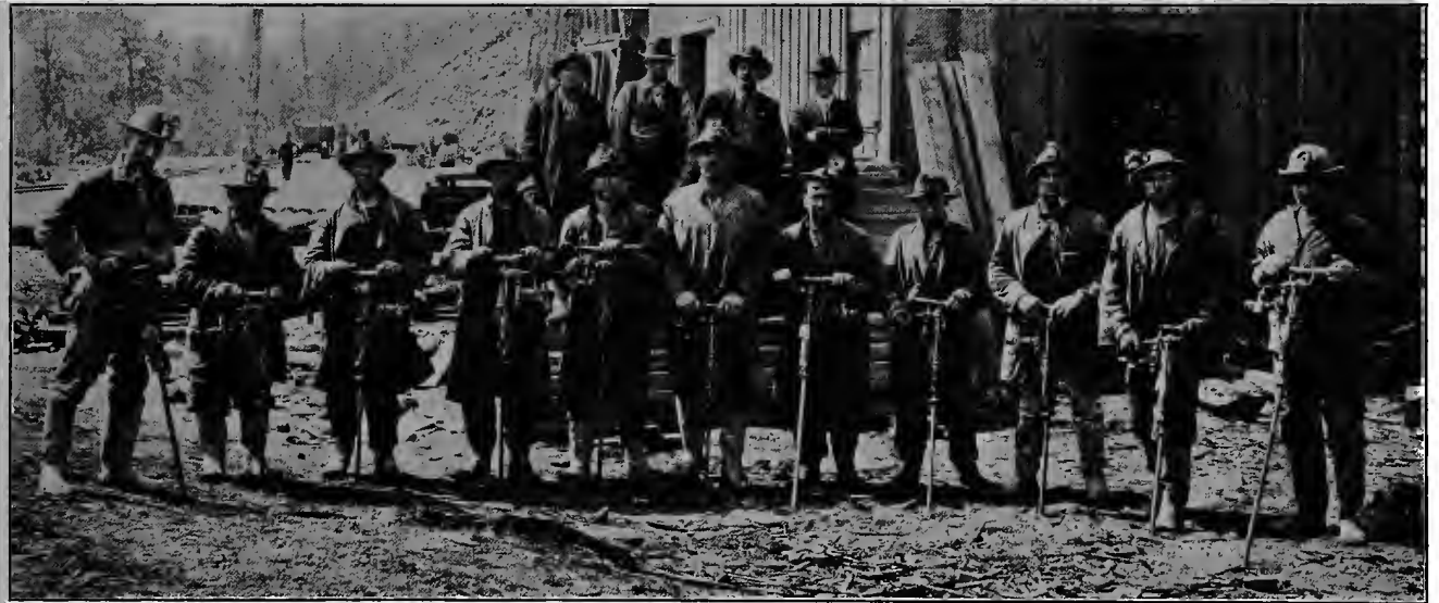
SHAFT CREW WITH HAND HAMMER-TYPE DRILLS USED IN SINKING SENECA SHAFT
