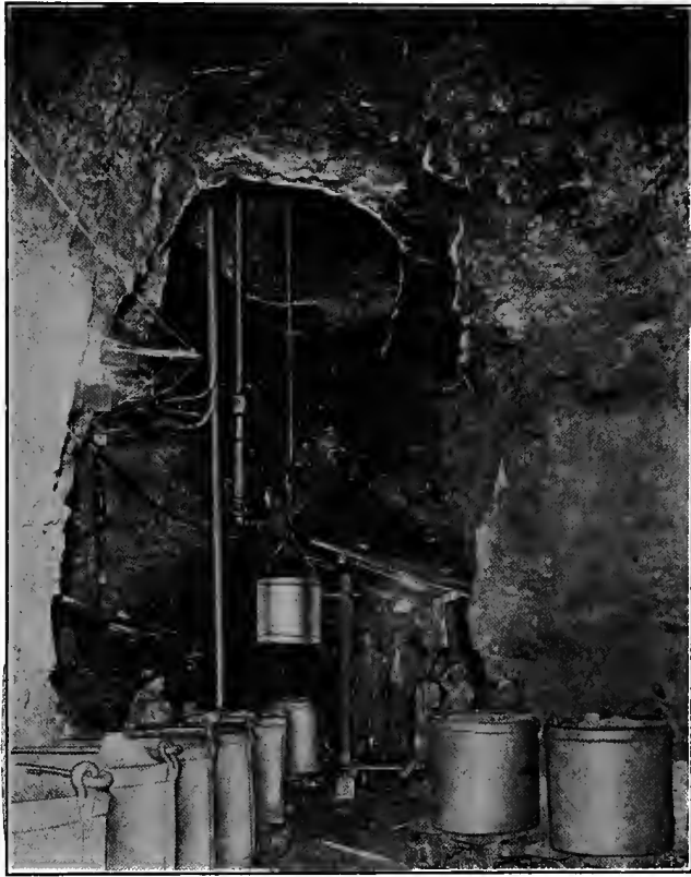
FIG. 10. HOISTING FROM A JOPLIN SHAFT STATION
