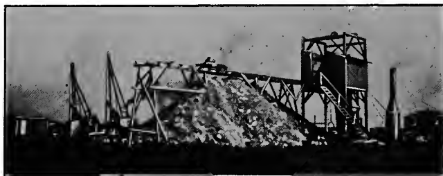
FIG. 12. DRILLING AND SHAFT SINKING NEAR PICHER, OKLA.
