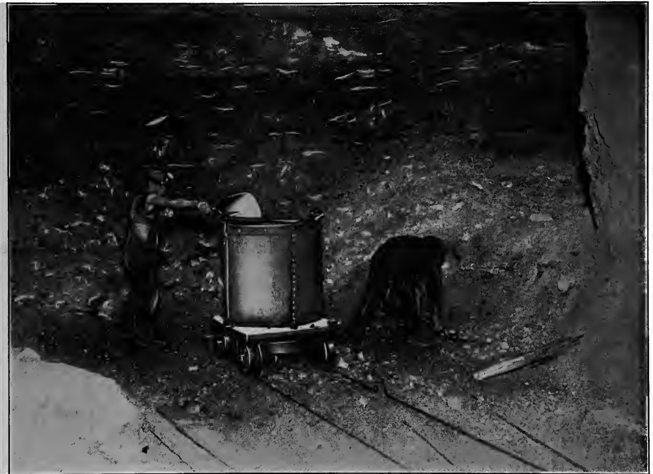
FIG. 13. SHOVELING CREW CLEANING UP A STOPE IN THE JOPLIN DISTRICT
