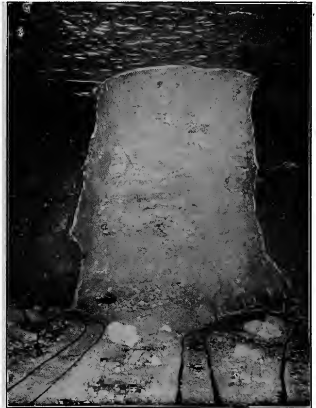
FIG. 11. CUTTING AROUND A PILLAR FROM TWO STOPES
