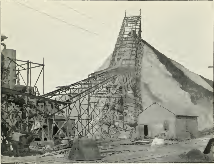
GREAT BOULDER TAILINGS ELEVATOR.
