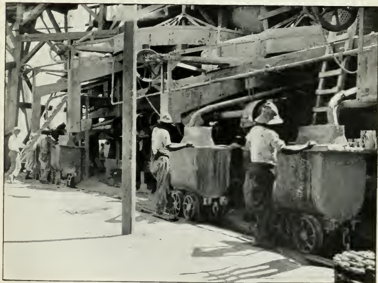
DRAWING OFF CONCENTRATES FROM PANS.
