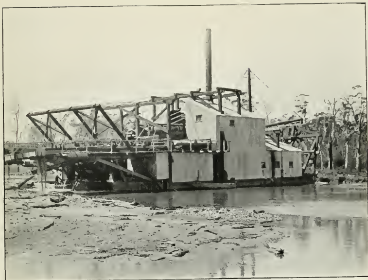
RINGAROOMA BUCKET DREDGE.
