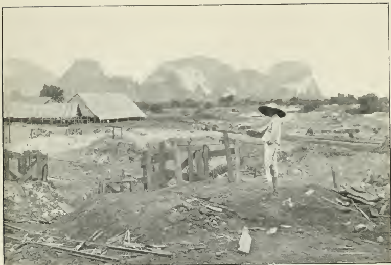
SUBSIDED WORKINGS, TAMBUN MINE, PERAK.
