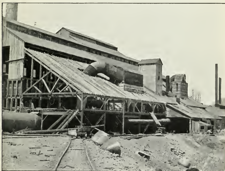
LARGE SMELTING FURNACE, DOMINION COMPANY.
