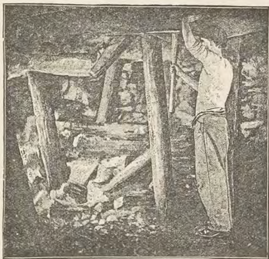
SUPPORTS FOR THE ROOF.
