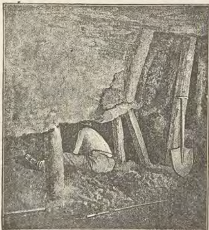
A DEEP UNDERCUT.
