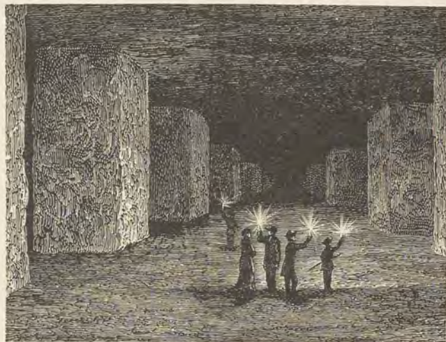
INTERIOR OF SALT MINE.
