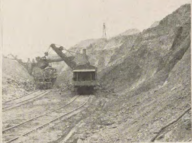
Top, left: Worker in Manganese mine, Independence County. Top, right: Mining Tripoli, Hot Spring County. Bottom: Working gravel pit with steam shovel, Saline County.
