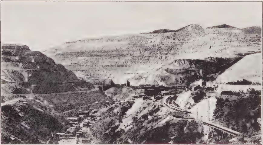
FIG. 804.—Open cut mine of the Utah Copper Company. Bingham Canyon, Utah. (Photograph by Underwood and Underwood.)
