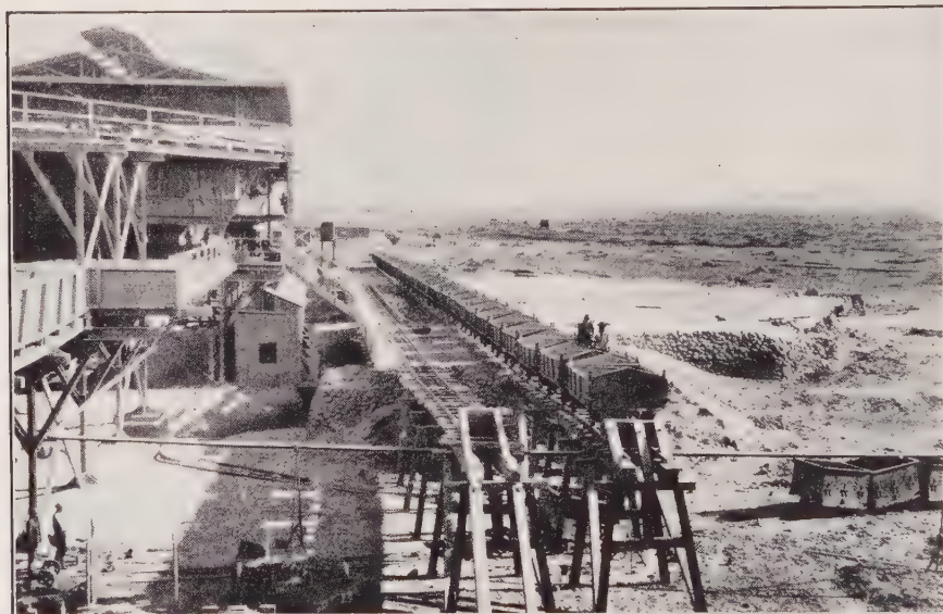
FIG. 808.—Cars loaded with crude sodium nitrate (caliche). Maria Refinery, Nitrate Field, Chile.
