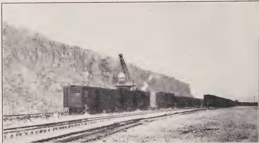
FIG. 812.—Loading sulphur. Texas Gulf Sulphur Company, Gulf, Texas.
