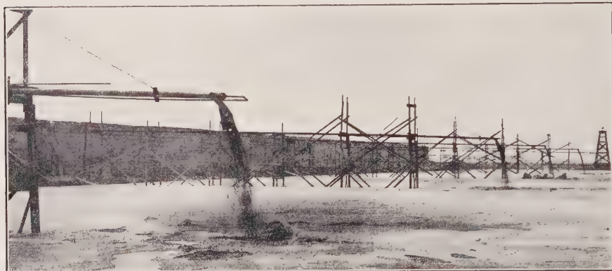
FIG. 492.—Sulphur discharge into vats by the Frasch method. Texas Gulf Sulphur Company, Gulf, Matagorda County, Texas.
