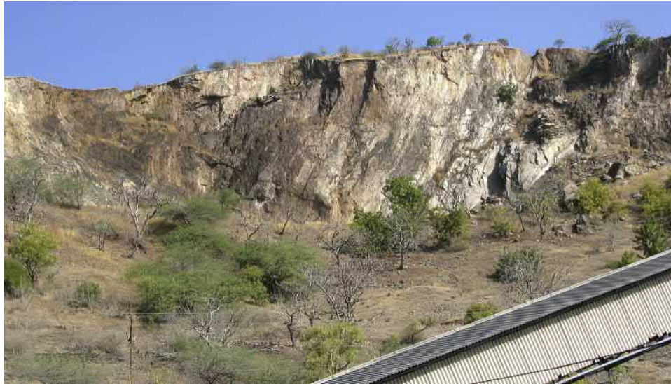
FIGURE 14.3 Surface subsidence from operating underground zinc-lead open stopes without any loss of life or material.
