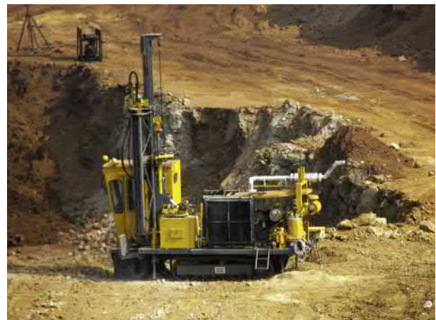
FIGURE 12.29 Compact crawler chain-mounted pit drill in operation at Sukinda chromite mine in India, to drill 5–10 m bench height and for easy movement to hole sites.
