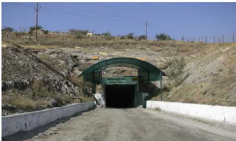
FIGURE 12.9 Mine entry systems through decline or ramp at a slope of up to 1 in 9 with fastest development to the bottom-most levels and suitable for earth-moving machinery and heavy-duty dumpers.
