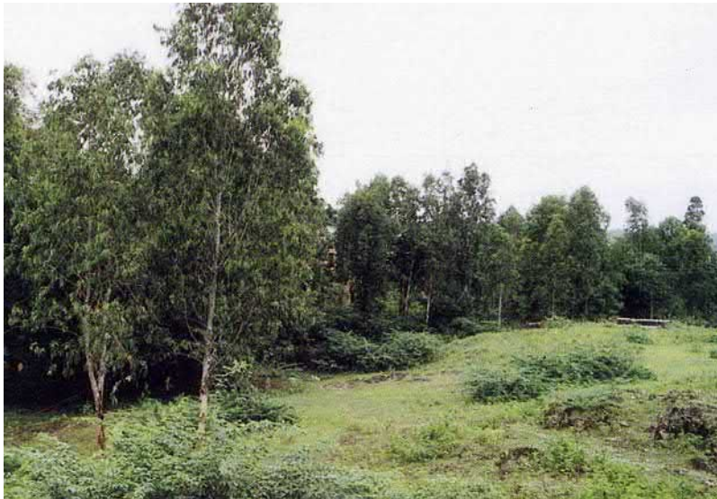
FIGURE 14.14 Plantation of vetiver grass and tall shady eucalyptus trees (Myrtaceae family) over abandoned old tailing dam at Zawar Group of mines, India.
