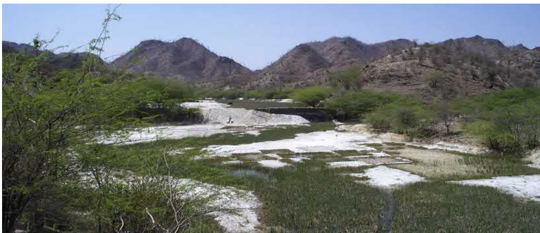
FIGURE 13.51 A panoramic view of a tailing dam in a hilly terrain that would eventually be filled over time, and rehabilitated by vegetative stabilization.
