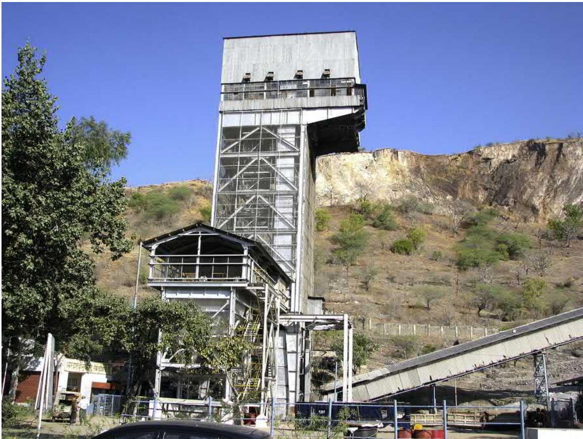
FIGURE 12.10 Main shaft with steel structure and conveyor belt at right-hand corner for ore transfer to mineral-dressing plant at Mochia Mine, Rajasthan, India.
