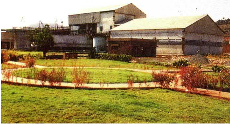
FIGURE 14.1 Reclaimed land used for building a zinc smelter at Visakhapattanam, India.
