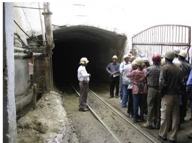
FIGURE 12.7 An adit—horizontal entry above the valley level to reach the orebody at optimum distance for underground mining at Zawar Mala, India.
