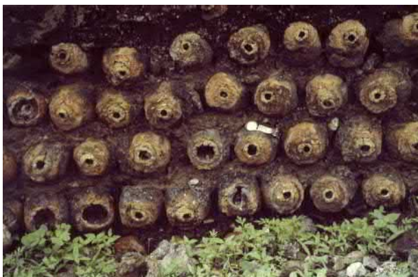
FIGURE 4.7 Ancient smelting retorts reused for the walls of a living shelter in the mining township at Zawar, India.
