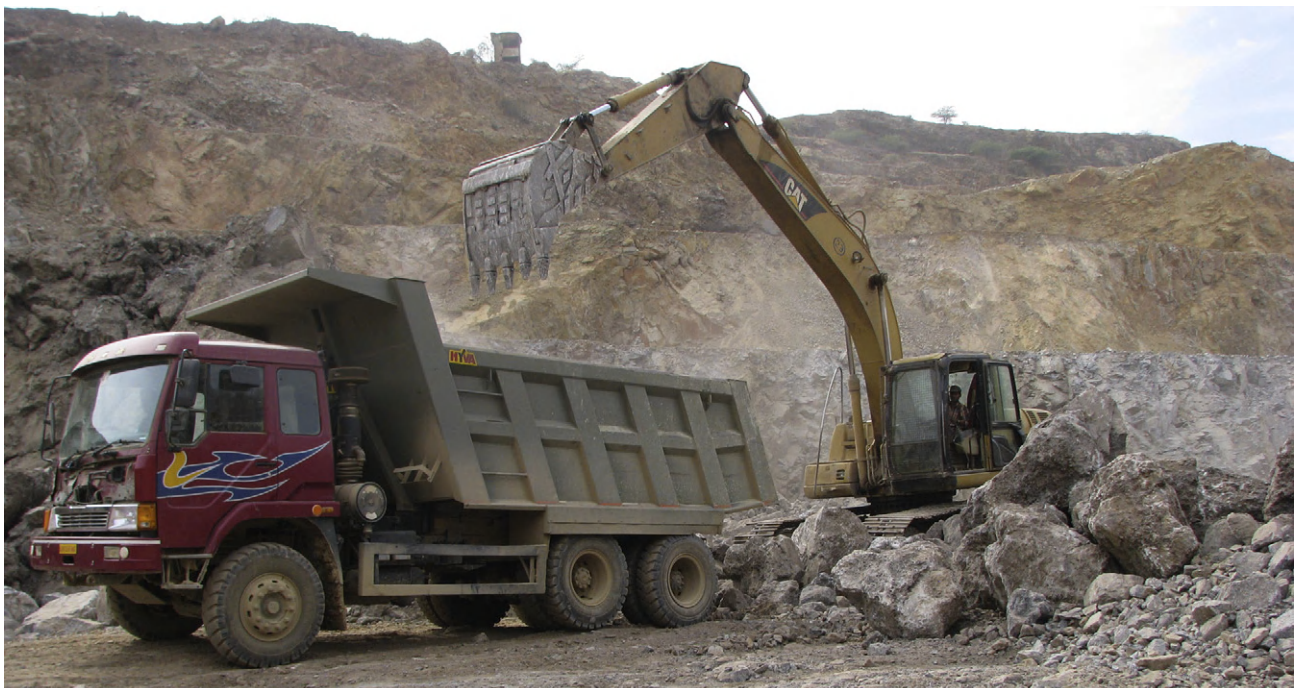
FIGURE 11.39 Hydraulic shovel loading and 85 t Haulpac dumper at Jhamarkotra rock-phosphate open-pit mine, Rajasthan (December 2008).
