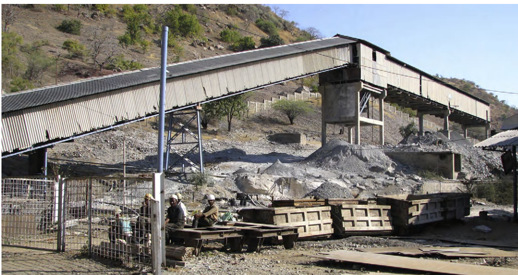
FIGURE 12.3 Close conveyor system (top) transporting ROM ore automatically unloaded from shaft cage to bin and interim stockpiles in the right with chutes at the bottom for auto-feeding to mineral process plant.
