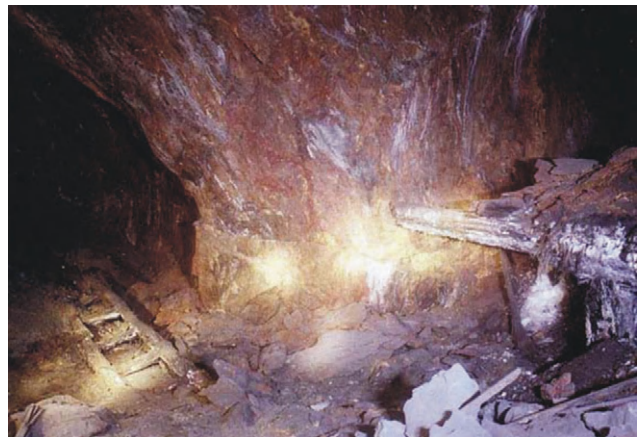
FIGURE 3.3 Ancient underground mining in rich zinc orebody at a depth of 172 m from surface. The arching of stope chamber evidenced high engineering skill. The wooden ladder (left) and platform (right) are still at abandon work site. Radiocarbon age dating indicates 3000 years from now at Rajpura-Dariba Mine, India.
