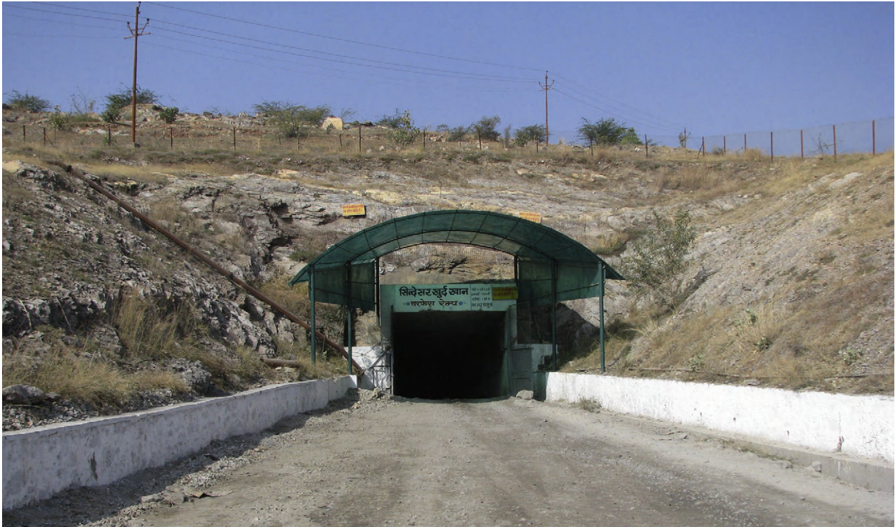
FIGURE 11.9 Mine entry systems through decline or ramp at a slope of up to 1 in 9 with fastest development to the bottom most levels and suitable for earthmoving machineries and heavy-duty dumpers at Sindesar Khurd Mine, India.
