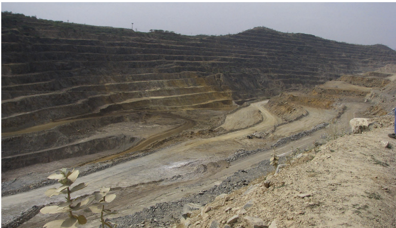
FIGURE 11.6 View of Jhamarkotra rock-phosphate mine with haulage road and series of overburden benches. The mine is planned for 7 km long, 700 m wide and 280 m ultimate open-pit limit at 2 Mt ore and 16 Mt overburden waste per annum capacity (December 2008).
