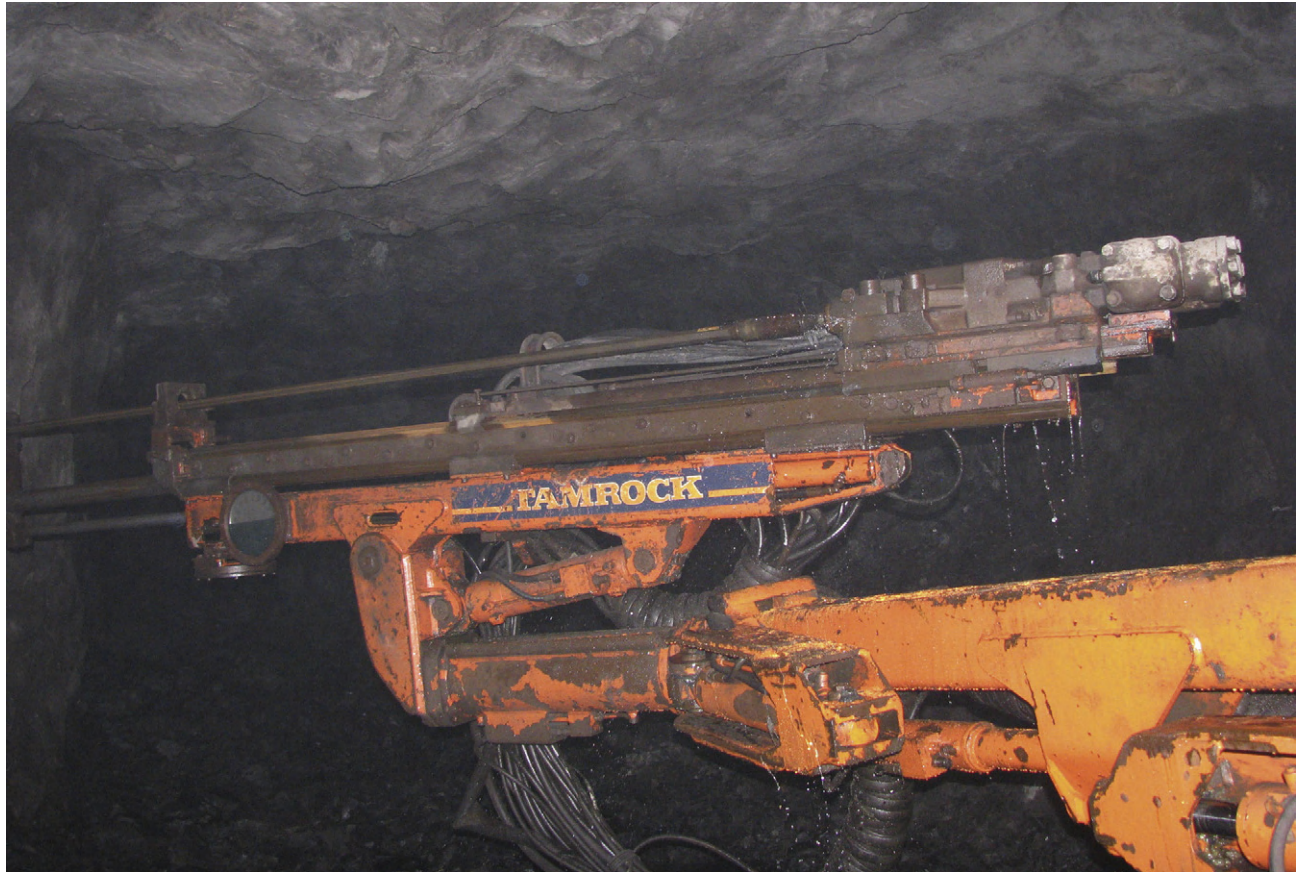
FIGURE 11.32 Close view of single-hand operator face drilling by Tamrock Single Boom electric-powered jumbo drill with straight 14 ft steel feed operation.
