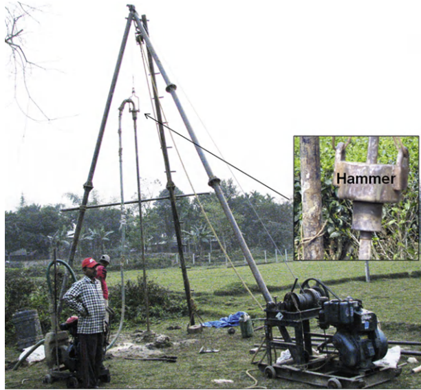
FIGURE 7.2 Percussion drilling in operation for rock quality and quick target test for mineral occurrences at low cost and time. The hammer is detailed in the inset.
