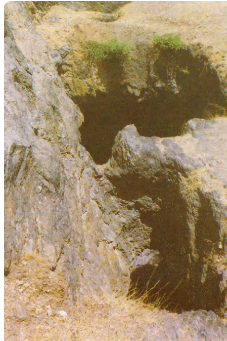
FIGURE 3.2 Ancient entry system to underground mine at greater depth with orebody plunge to northeast at Rajpura-Dariba copper-zinc-lead-silver mine, India.
