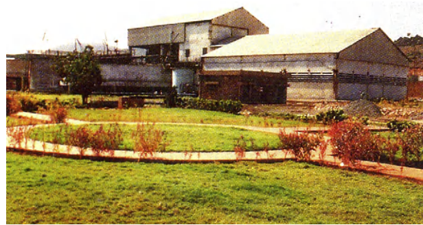
FIGURE 14.1 Reclaimed land used for building zinc smelter at Vishakhapatnam, India.
