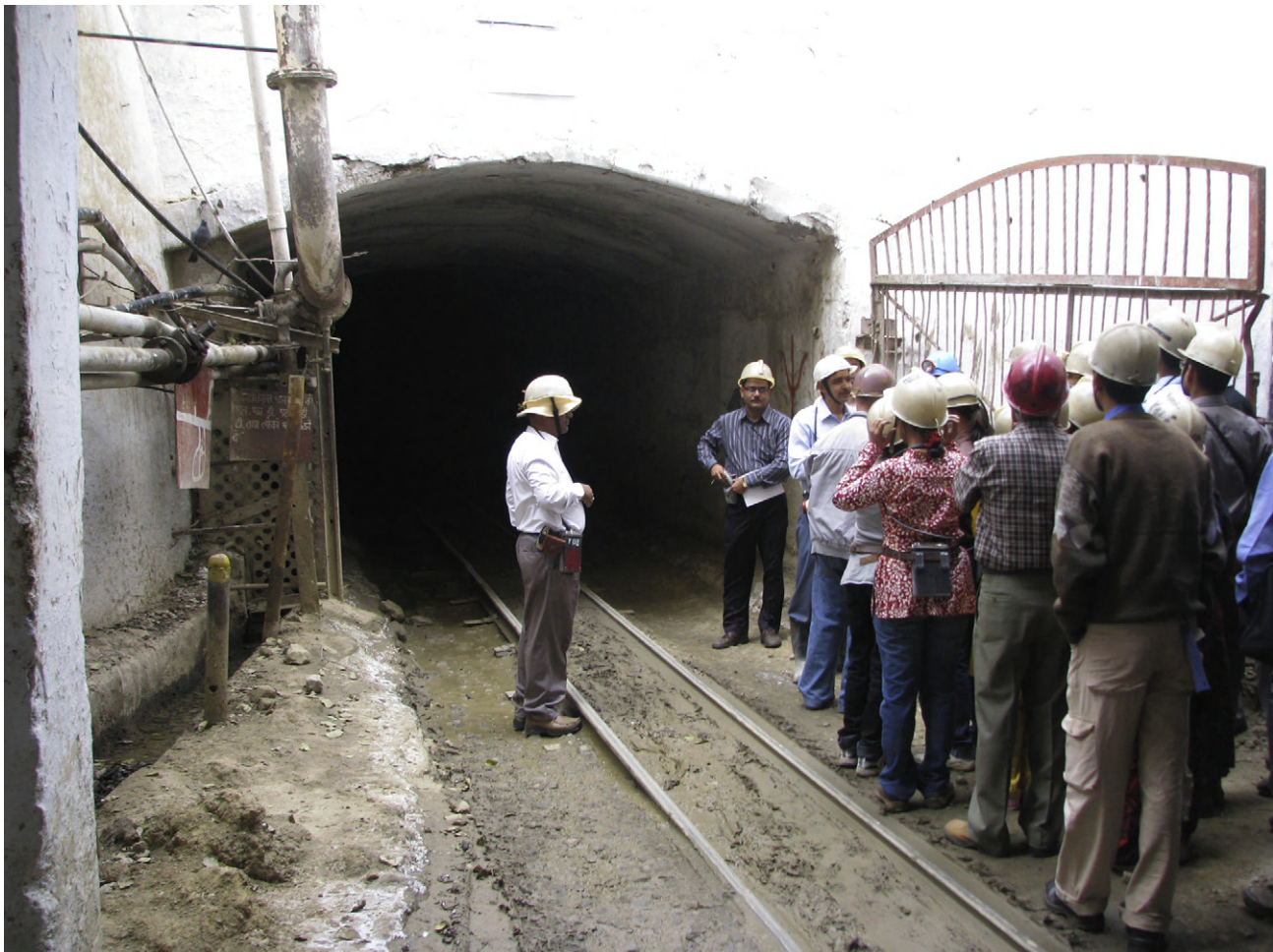
FIGURE 11.7 An adit—horizontal entry above the valley level to reach the orebody at optimum distance for underground mining at Zawarmala, India.
