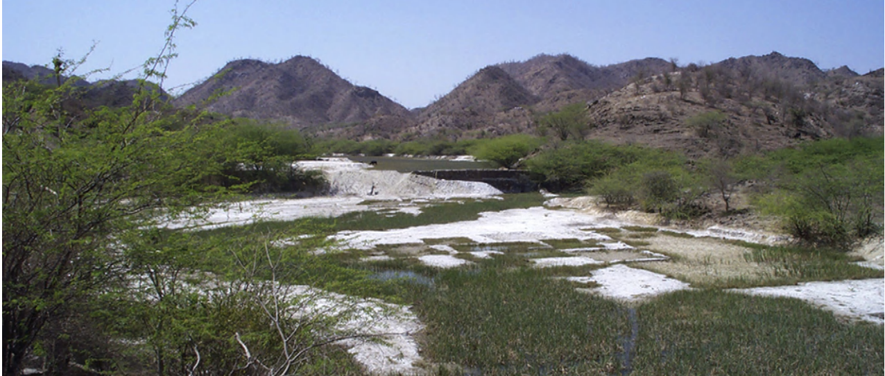
FIGURE 12.53 View of tailing dam in a hilly terrain that would eventually be filled over time and rehabilitated by vegetative stabilization.
