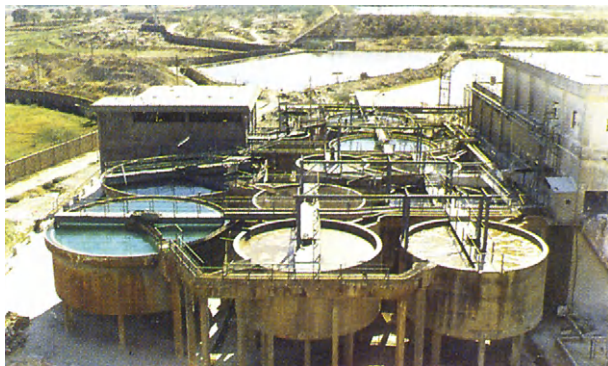
FIGURE 14.13 Effluent treatment plants to recover metals and recycling of water for industrial uses, Rajasthan, India.
