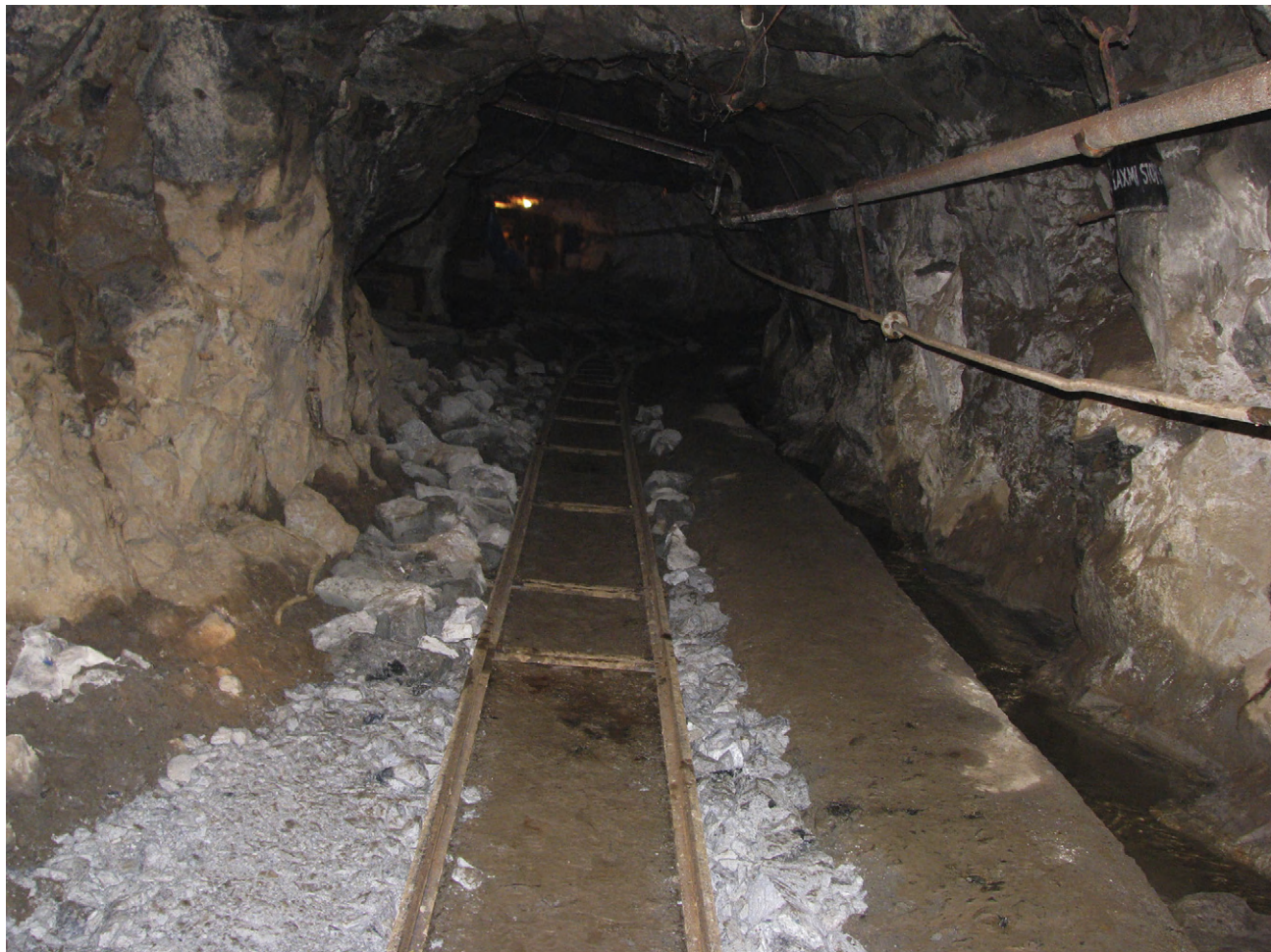
FIGURE 11.14 View of a main crosscut starting from the central main shaft to the orebody at Boula-Nausahi chromite deposit and operates as main production haulage (December 2009).
