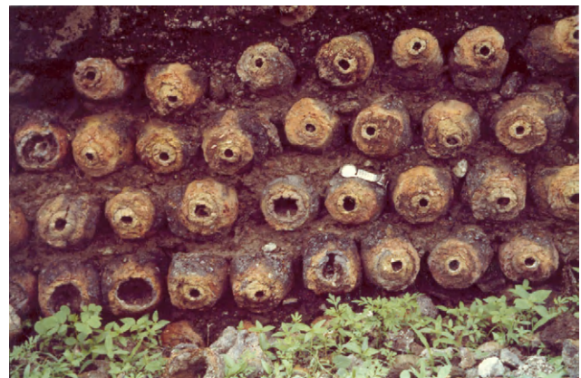
FIGURE 3.7 Ancient smelting retorts reused for walls for living shelter in the mining township at Zawar, India.
