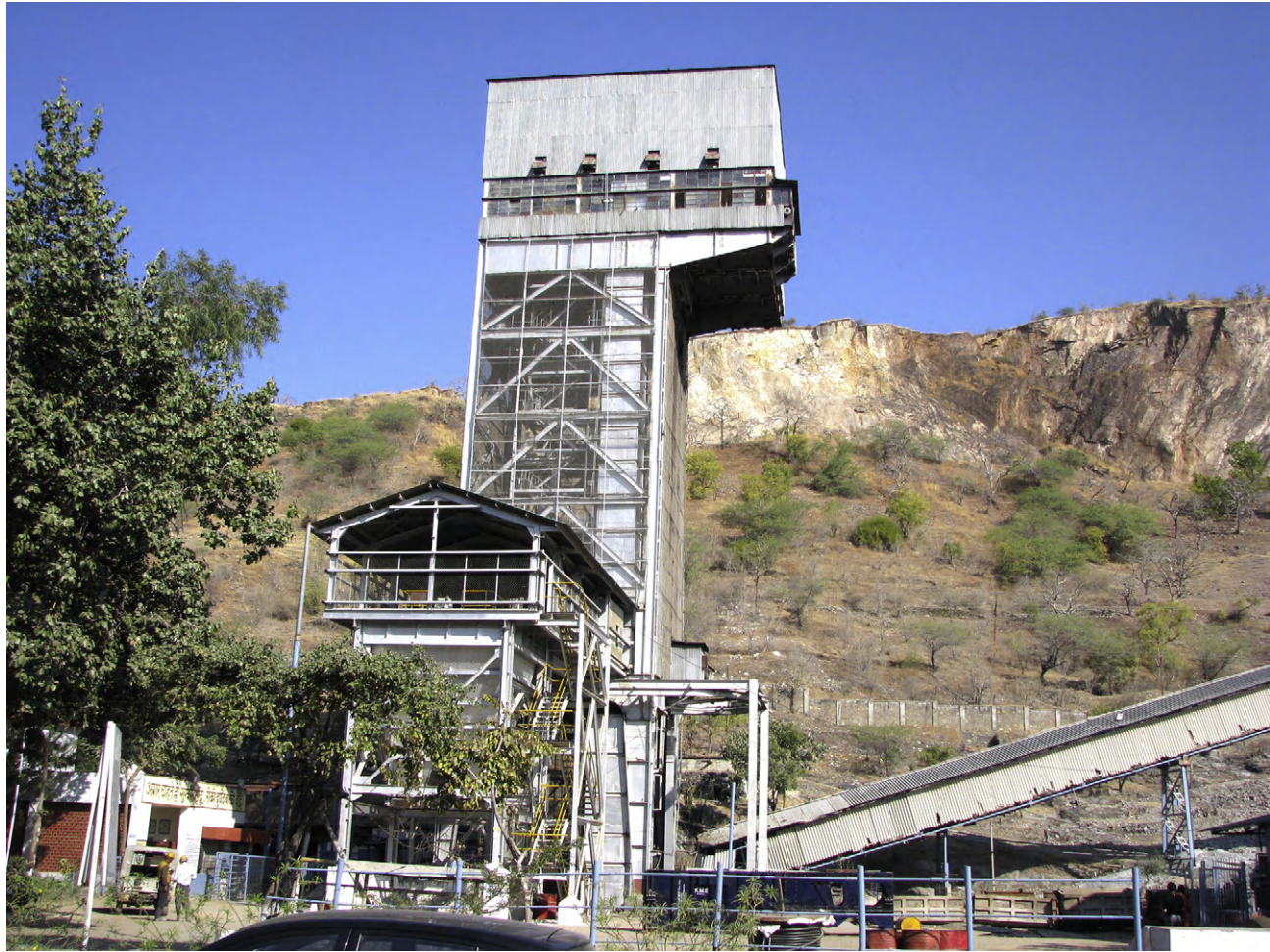
FIGURE 11.10 Main shaft with steel headframe and other structure in the center, and conveyor belt at right hand corner for ore transfer to mineral dressing plant at Mochia Mine, Rajasthan.
