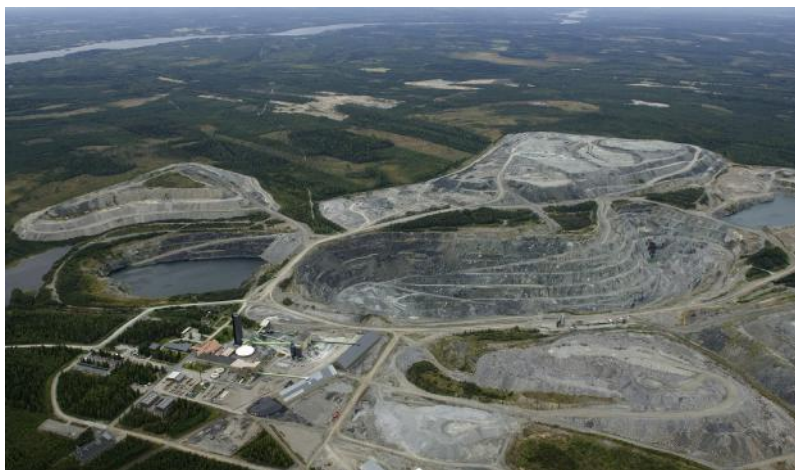
FIGURE 3.4.11 Aerial photograph of the Kemi Mine looking north.
