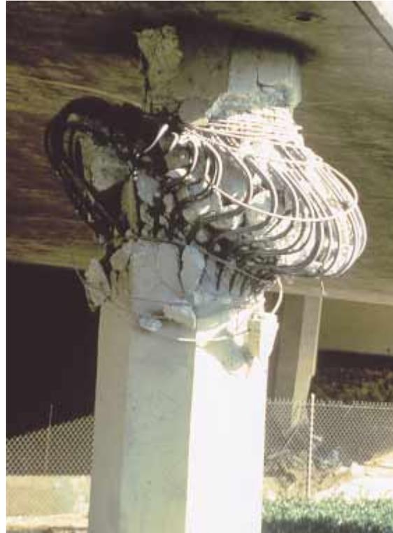
**Figure 1–12** Earthquake-resistant design allowed this bridge support to rupture during the 1994 Northridge, California, earthquake, but prevented total collapse of the bridge. (Earthquake Engineering Research Institute)
