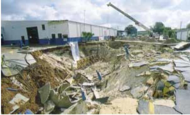
**Figure 15-11** A dropping water table caused subsidence and structural damage in Jacksonville, Florida. (Wendell Metzen/Bruce Coleman, Inc.)
