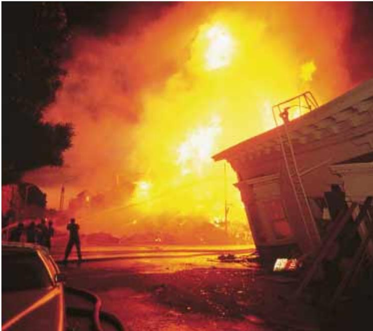
**Figure 10–17** Ruptured gas and electric lines often cause fires during earthquakes in urban areas. This blaze followed the 1989 San Francisco earthquake. (Lysaght/Gamma Liaison)
